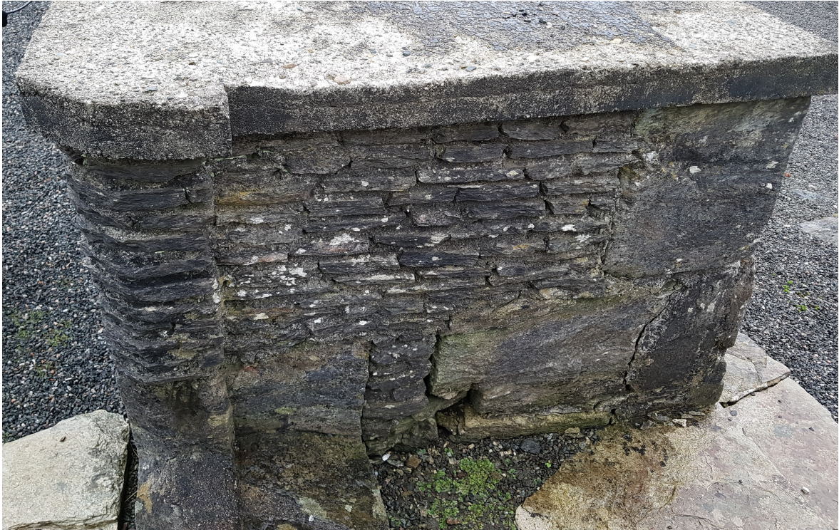
FIGURE 2.13: The workshop wall viewed from its side.
