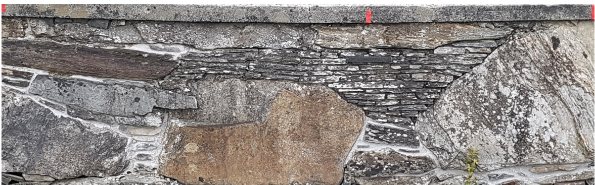
FIGURE 2.15: The kitchen wall.
