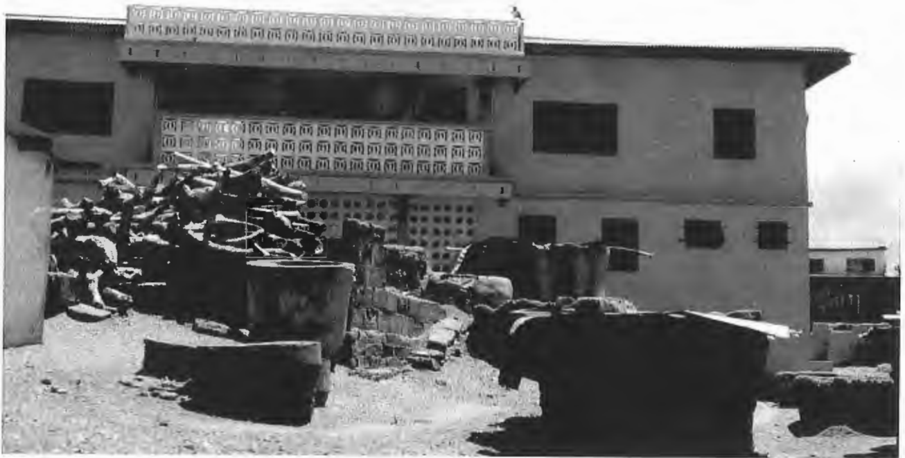
Photo 17. The late Esi's house; painted for the funeral and with the cemented smoking ovens in front, still inactive after her death. But piles of firewood indicate plans of further fish smoking activity.
