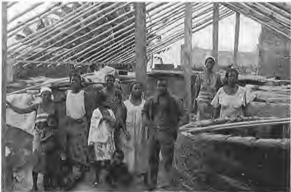
Photo 12. Members of a matrilineage cooperate in the building of a smoking-shed over circular mud ovens at ruins of Fort Nassau.
