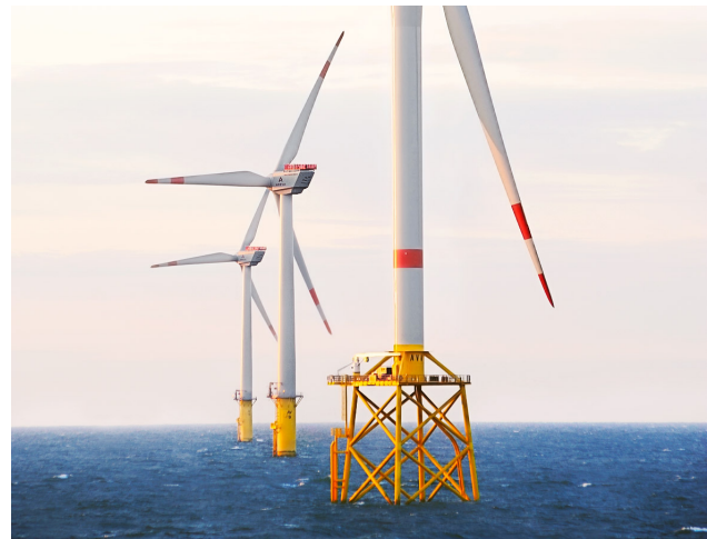
(b) Alpha Ventus turbines and foundations: Servion turbine with jacket foundation in front, and Adwen turbines with tripod foundations in the back, figure from [130].
