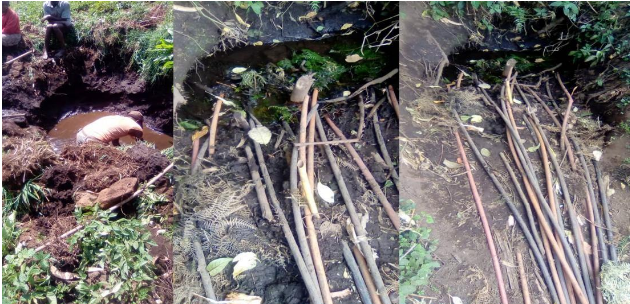
Picture 5.6: How water catchments are exploited for irrigation. Source: fieldwork 2021 The First picture to the left showing farmer digging to increase the depth of water table, second and third pictures showing how tens of rubber pipes are being placed in water catchment to channel water to the plots with the use of canon pipes and fen plants to filter the dirt or mud from getting into the pipes.
