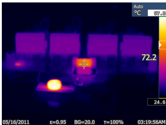
(a) Overview of the converter
