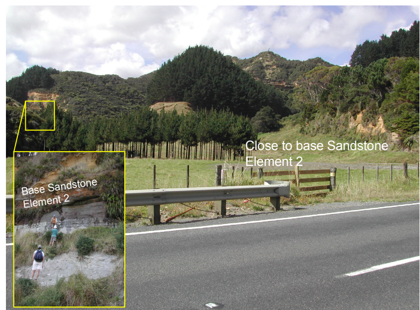
Figure 3.14 Base of Sandstone Element 2 as exposed in lower part of Rapanui Valley, State Highway 3 in front, see Figure 3.9 for location.
