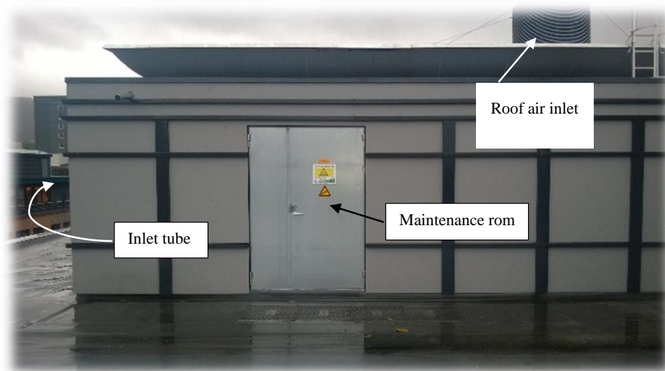
Figure 14. At the roof of the office building. Picture illustrates the entrance door to the maintenance room and at the right top it is possible to spot part of the ventilation systems air inlet.
