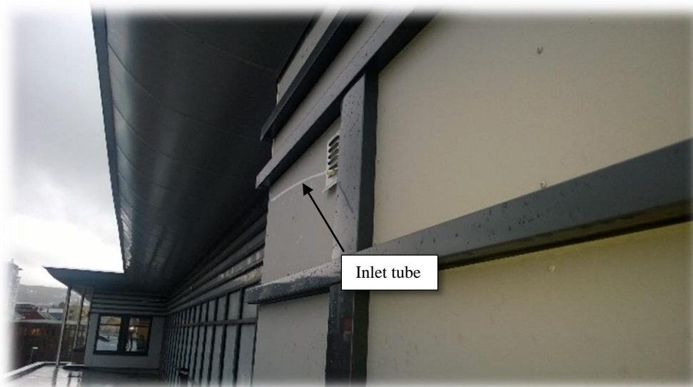
Figure 15. Sampling at the roof of the office building, near the roof-air inlet as illustrated in Figure 11 and Figure 7.
