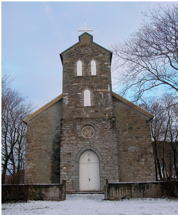
Figure 6. The west front of Tjøtta church as it appears today after the last rebuilding finished in 1851. Soapstone ashlars from the medieval church are visible in the wall together with rubble stone. (Photo: B. Berglund).
