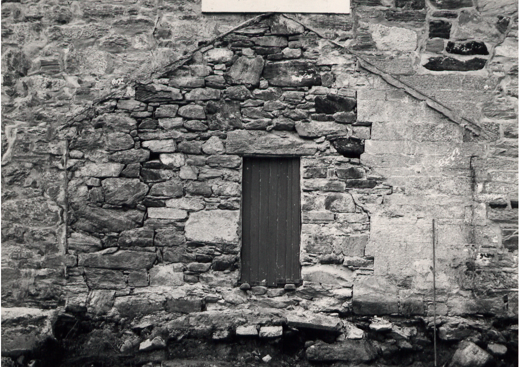
Figure 8. The outer east wall of the chancel in Brønnøy church. The photograph from 1960 shows that a section of the medieval wall with soapstone ashlars is preserved. (Photo: E. Høvding. ©The Directorate for Cultural Heritage, The Archive).
