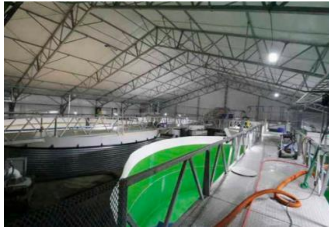
Figure 2.2: The large hall at Hardingsmolt facility with all the 12m tanks. The closest tank is empty at the time when the picture was taken. Bridges to walk on can be seen right over the tanks for the farmers to have an easy access to each of the tanks (Heima, 2016).
