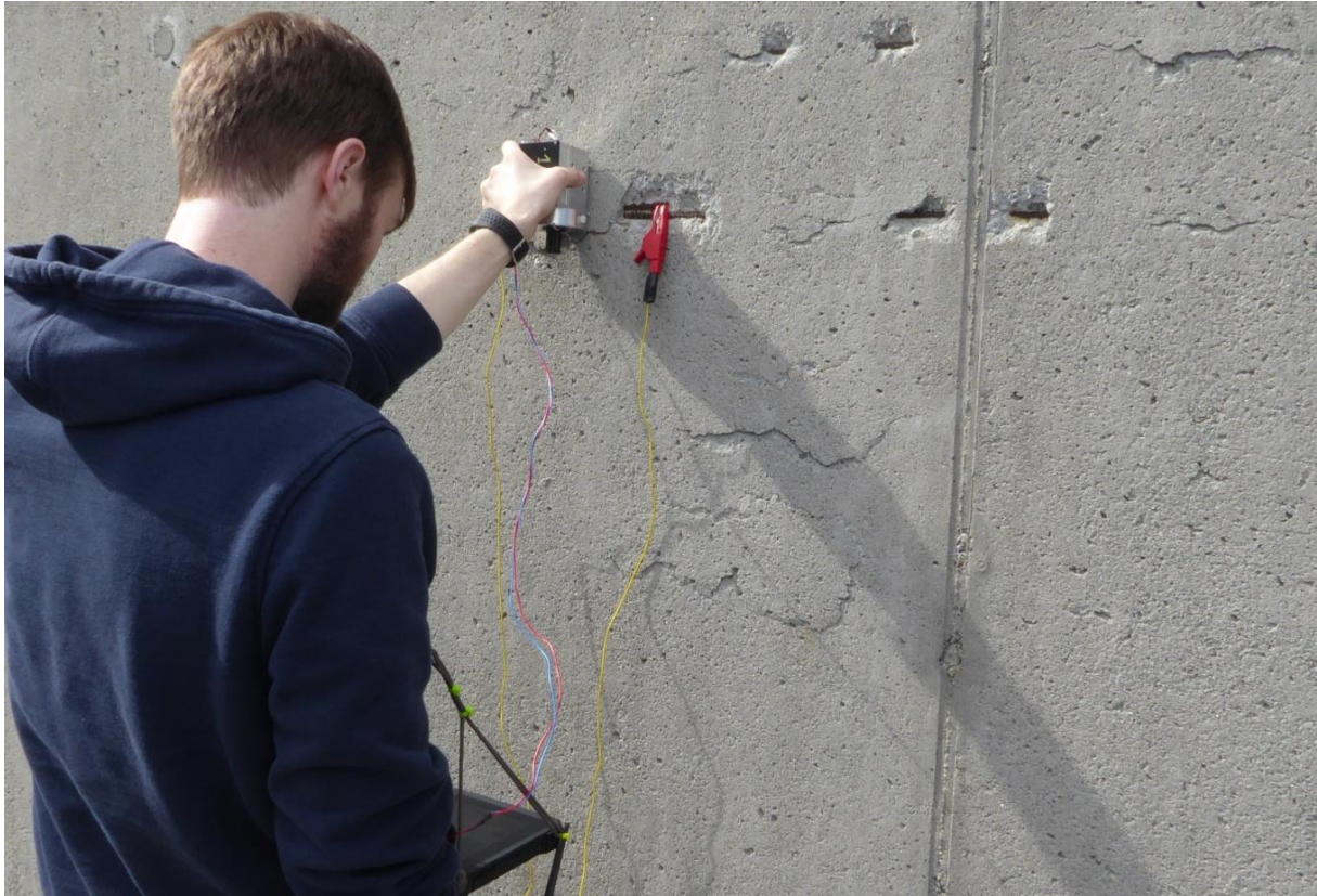
Figure 15: Early field test with the FKP, showing how it may be used. The instrument is powered by batteries and is controlled via Bluetooth from a tablet. Yellow wire used to ground the FKP to an exposed rebar.
