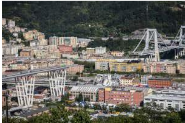
Figure 1: Genoa bridge collapse, August 14 th , 2018. Corrosion is a possible cause. [1]
