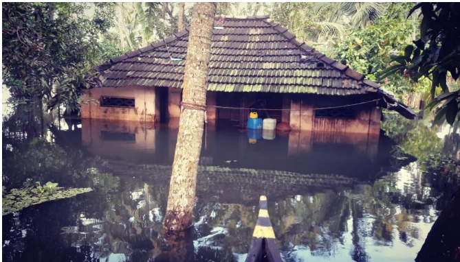
Photo 7. Image of floods.
