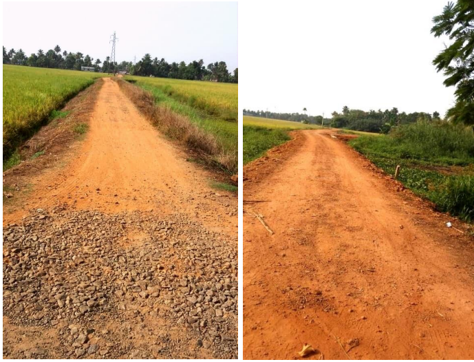
Photos 14 and 15. Road built cutting across paddy fields.
