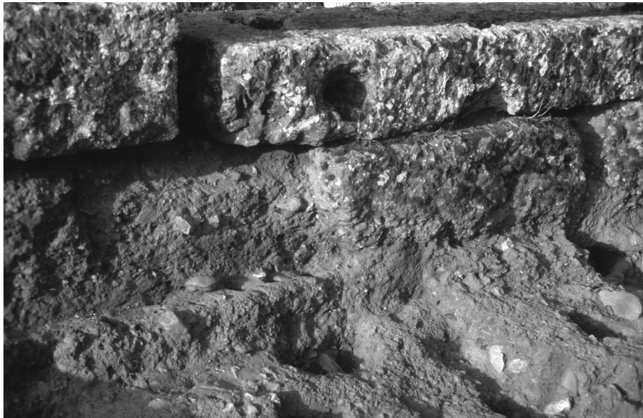
Figure 15. The southern Archaic colonnade foundation, supported at some points by other blocks (right), elsewhere only by debris (left). (Photo: E. Østby)
