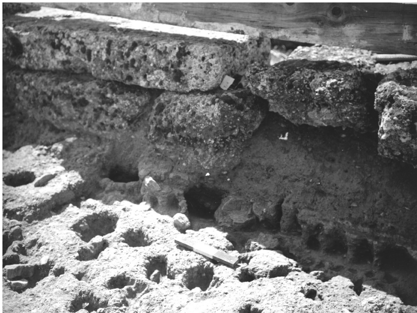
Figure 58. Below the Archaic stone foundation the clay structures of the southern wall of Building 2 can be seen, with indents from reeds inside the wall (extreme right) and surface with postholes in front. Seen from north-west. (Photo: Nordquist)
