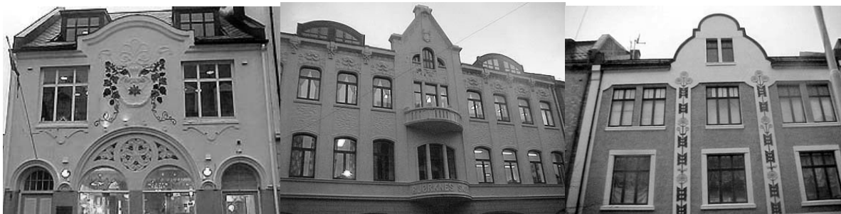
Figure 22. Jugend buildings in Ålesund probably erected in Bergen cavity brick walls. Pictures from Globalnytt 3, Norsk nettskole: http://www.avsenteret.no/nettskolen/globalnytt/3/jugend.htm
