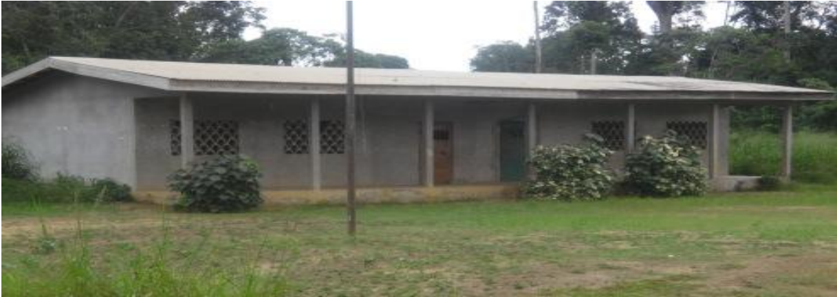
Photo 5.5 Classrooms at Bikondo
