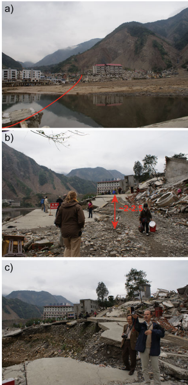
Fig. 9 Fault scarp in Beichuan, crossing the river with a 2.5 m uplift. a View towards SW, the old part of Beichuan with alluvial material in the foreground, the red line marks the continuation of the fault across the valley. b Surface rupture in Beichuan. The picture is taken towards the new part of town to the NE, at the same location as (a). Vertical uplift of 2–2.5 m was measured in Beichuan, as indicated with the red arrow . c Close-up of the fault scarp, where deformed concrete road blocks and rubble from collapsed buildings are visible
