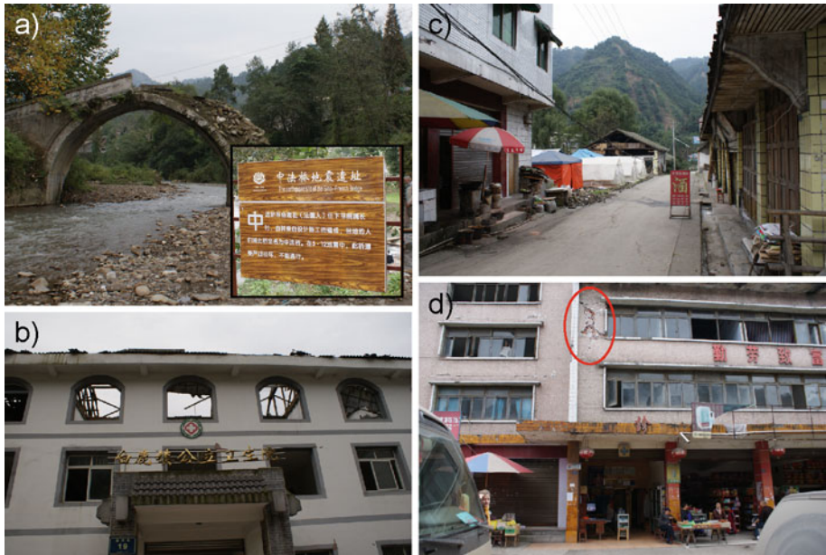
Fig. 6 Damage to structures in the city of Bailu. a Zhongfa Bridge crossing the river in Bailu. b City hospital, which suffered from roof collapse. c–d Main street of Bailu, where large cracks are visible in the house walls. Temporary shelters and tents are visible in the background of c
