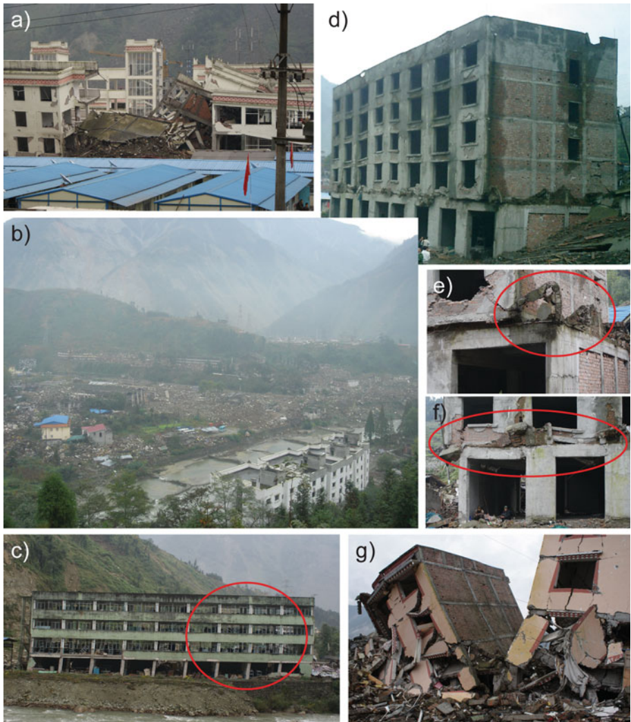
Fig. 4 Building damage at Yingxiu Town of Wenchuan County. a Xuankou Middle School, shelter buildings are visible in the foreground. b Overview of Yingxiu where ca. 80% of the city's buildings collapsed during the earthquake. c Factory building with clearly tilted columns. d–f Six-story RC-brick infill building which suffered a single story collapse of the second floor. g Partial collapse of residential buildings
