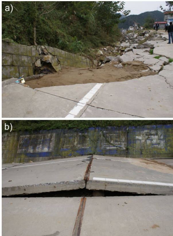
Fig. 20 a Evidence of liquefaction, where the wall and road has sunk into the sand. b Buckling of concrete road blocks
