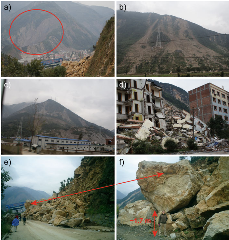
Fig. 17 Landslides and rock falls in Beichuan. a–c Landslide scarps visible on the steep mountain slopes surrounding Beichuan. Temporary shelters are visible in the foreground of (c) . d Landslide in the center of Beichuan, causing an apartment block to total collapse. To the right a building with no apparent damage is visible. e–f Large rock falls and boulders blocking the road to Beichuan, notice the huge size of the boulder in (f)
