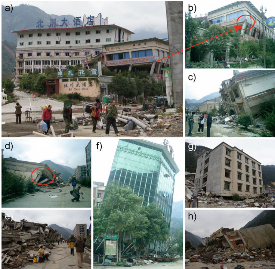
Fig. 10 Building damage in Beichuan County Town. a–b Bei Chuan Hotel suffered severe damage, as failure of the column beam joints, but sustained the ground shaking. The main building of the hotel is clearly tilted ( a ). c–e Main street of the newer part of Beichuan, with collapse of weak structures due to column failure. f–g Buildings suffering single story collapse of the first floor. h Toppled building due to ground failure
