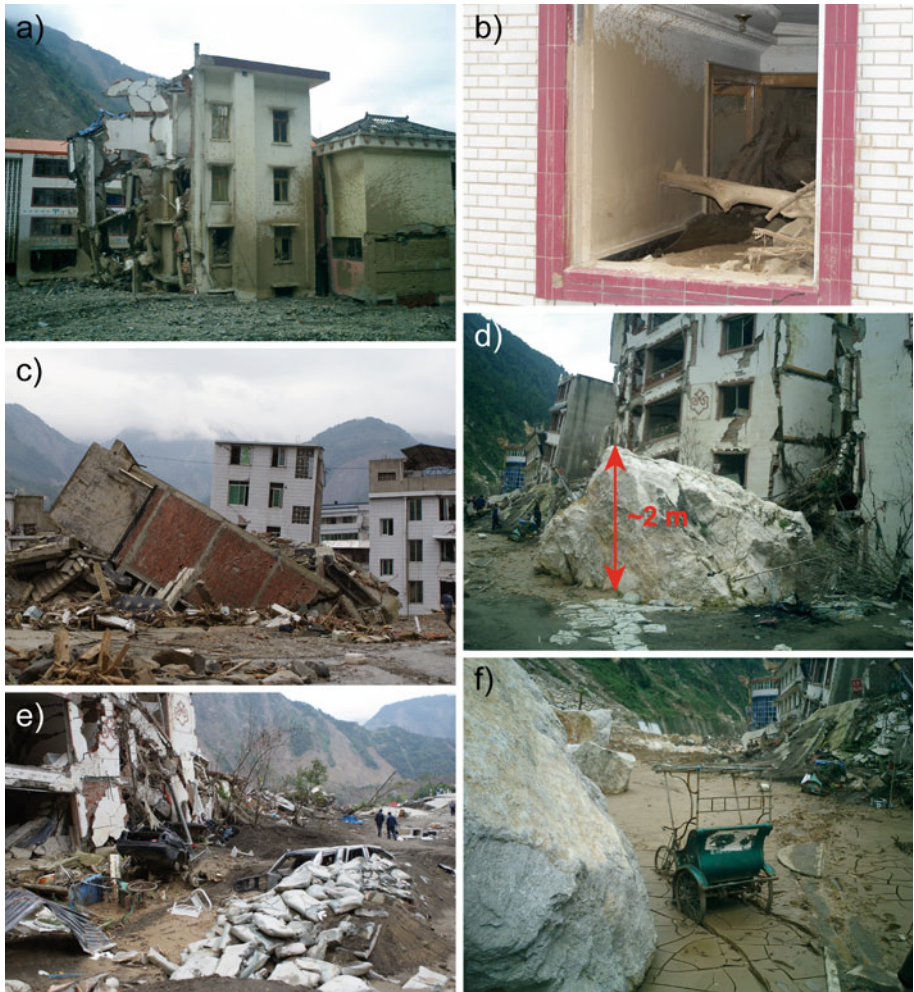
Fig. 19 Debris- and mudflow in Beichuan. a–b Splatter stains of mud on outer and inner walls of houses in the debris area verifying the strength of the event. c Toppled building in the old part of Beichuan due to ground failure during the ground shaking. d–f large boulders, cars and other objects stuck in the thick layer of mud and debris material. In d and e buildings with extensive damage due to strong ground shaking is visible
