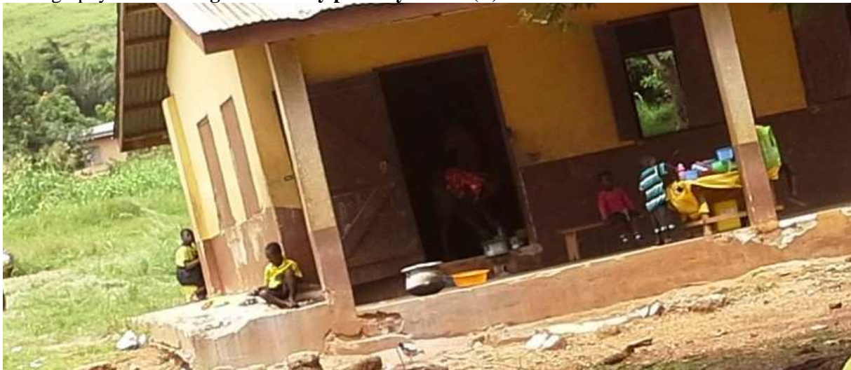
Photography 5.2 Building one used by primary school (B) and KG.
