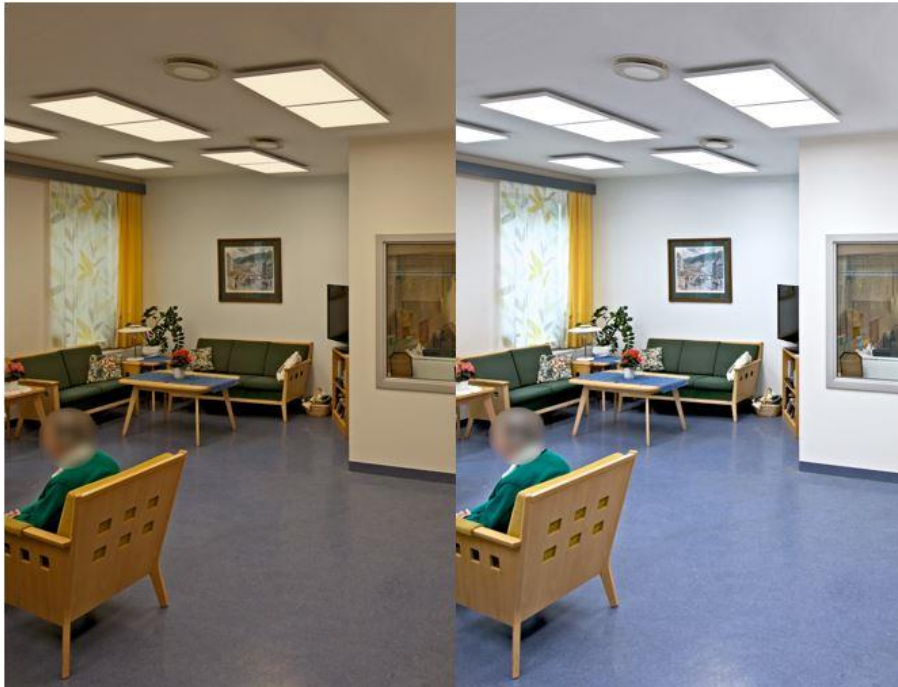
Figure 4: An illustration of the contrast between the spectral composition of standard light (left, 3,000 K) and the spectral composition used in the intervention (right, 6,000 K). The photos show one of the units in the intervention group. Source: Photos provided by Glamox, reprinted with permission.
