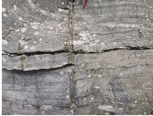
Figure 2.1: Rock exposure with fairly regularly oriented fractures of varying size.
