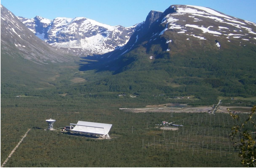
Figure 3.5: EISCAT facility at Tromsø. VHF (parabolic cylinder) and UHF (parabolic dish) radars are located in the lower left part of the photo. Photo taken from mountain Storforsaksla (North of the radar site), my first visit to Norway on July 06 2012.
