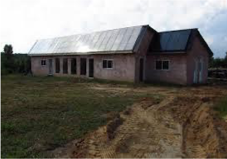
FIGURE 2- SOLAR PANEL ROOF AT LIVING ENERGY FARM
