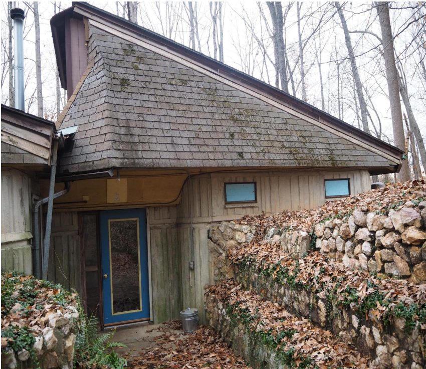
FIGURE 6- ENTRANCE TO DEGANIA—THE CHILDREN'S HOME-SCHOOLING HOUSE AND PREVIOUS DORM ROOM
