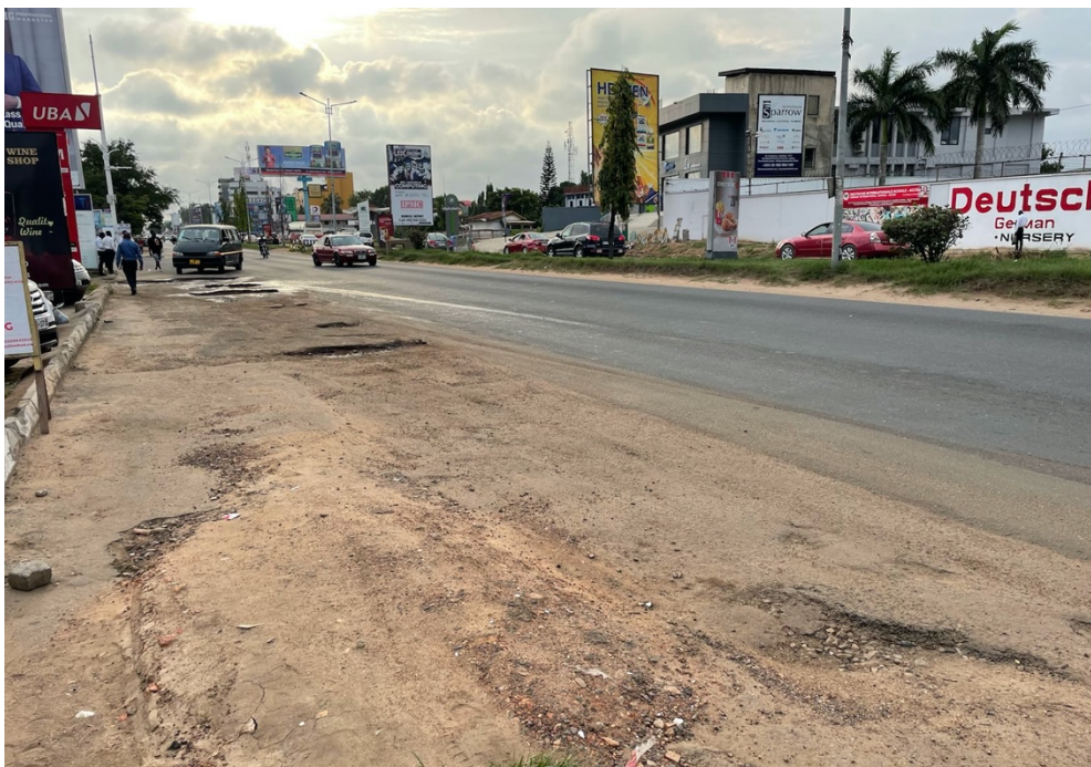
Figure 6: Decreasing quality of the road from center towards the side. Source: Fieldwork 27.09.2021
