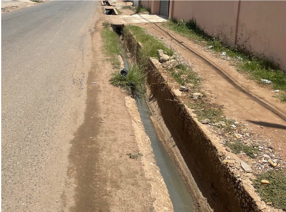
Figure 5: Wastewater channels that can be found on most roads in Accra. Source: Fieldwork 18.09.2021
