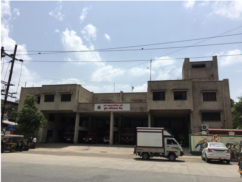
Figure 17: Mumbra Fire Station. P.C. Sumanya Anand Velamur
