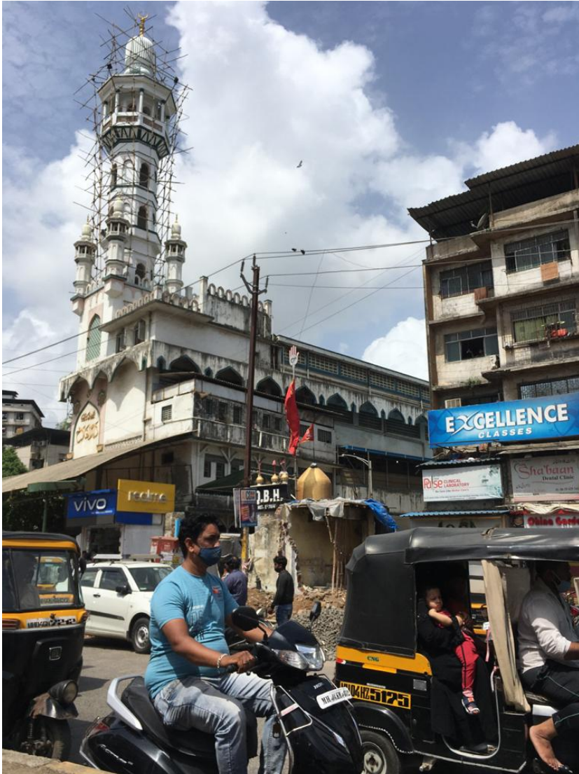
Figure 18: Darul falah mosque undergoing renovation. P.C. Sumanya Anand Velamur
