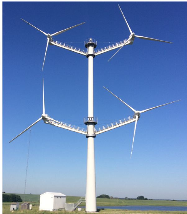
Figure 1.2: The Vestas 4R-V29 multirotor wind turbine. From [11].
