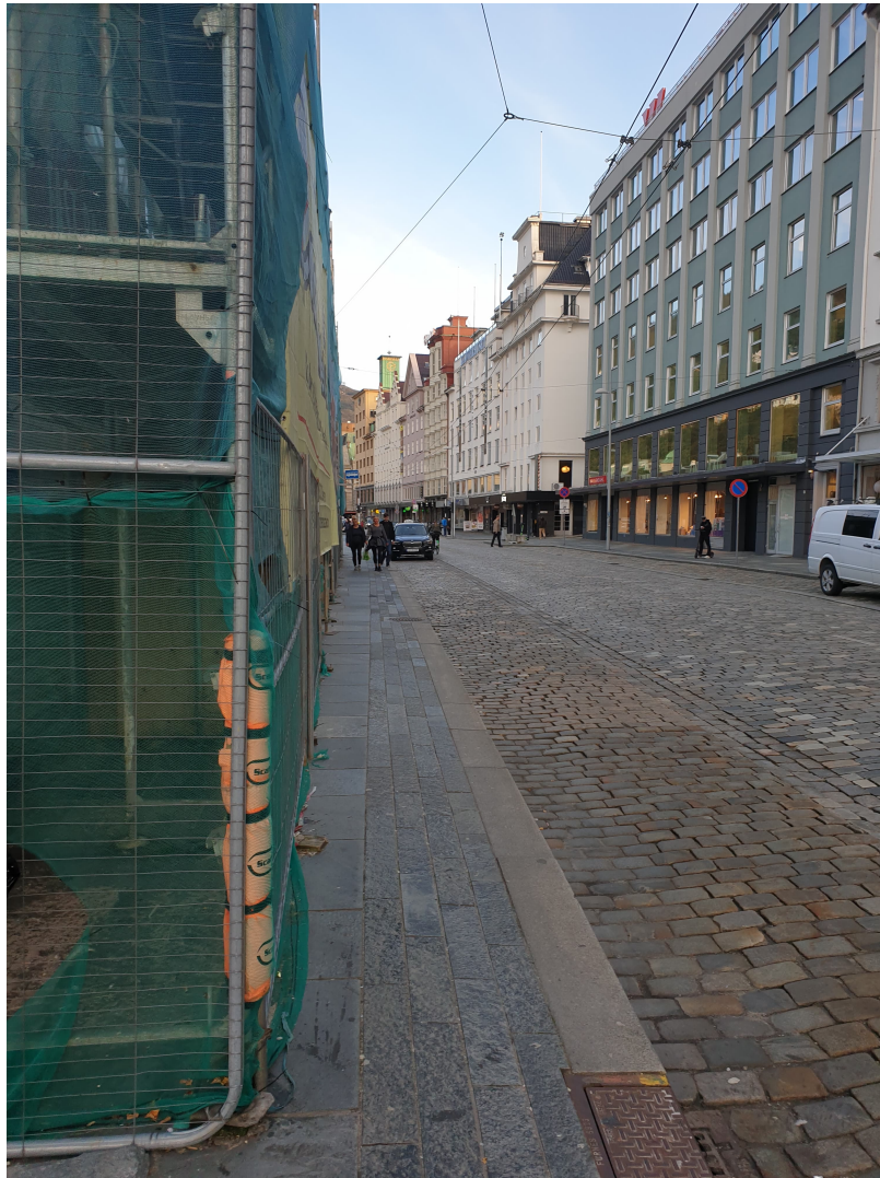
Figure 6.5: Constriction work making the path quite narrow
