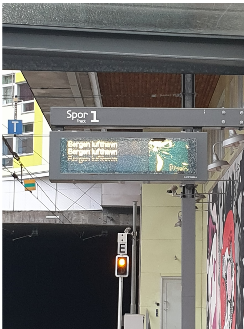
Figure B.1: The sign at the light rail stop was broken
