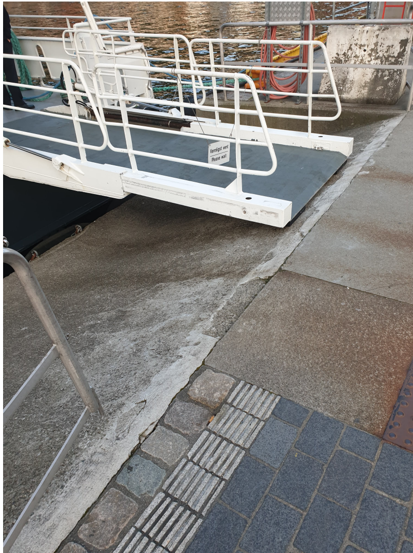
Figure 6.7: Depending on the sea level, the boarding ramp can be lower on the other ramp making it quite steep
