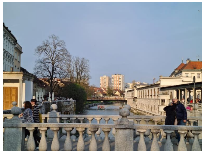
Bridges connecting the riverbanks
