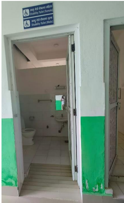
Figure 15: Disability-friendly Toilet of Nawalpur Primary Hospital
