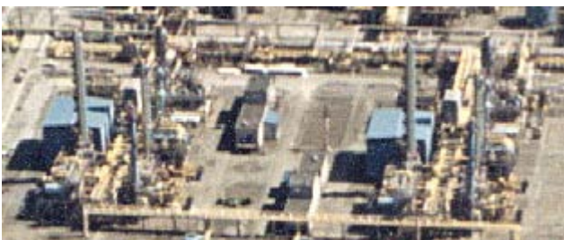
Figure 8 Statpipe processing trains
