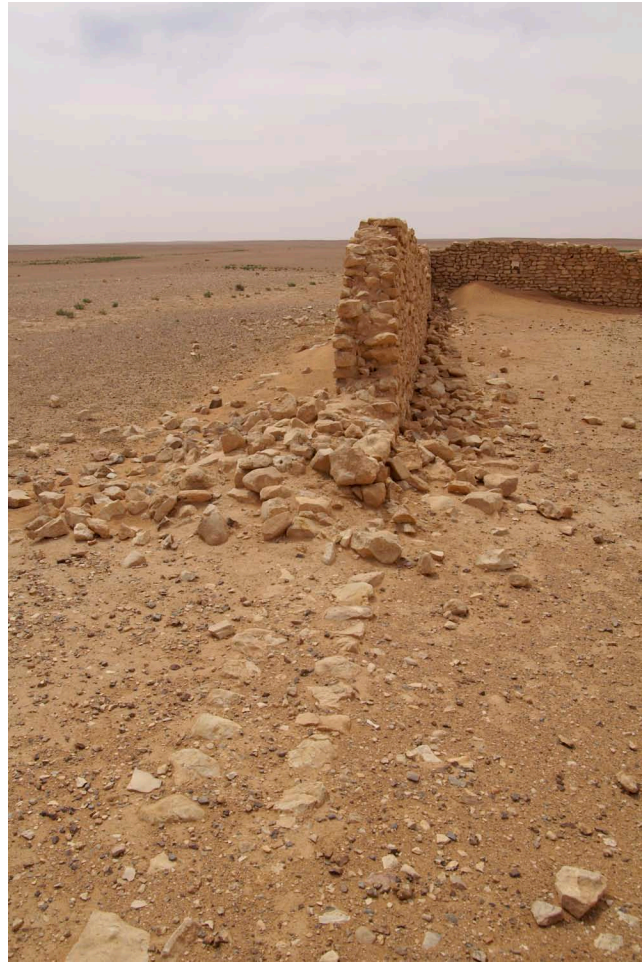
Modern abandoned building built of mud-built stonewalls. Joufar SE of Palmyra.
