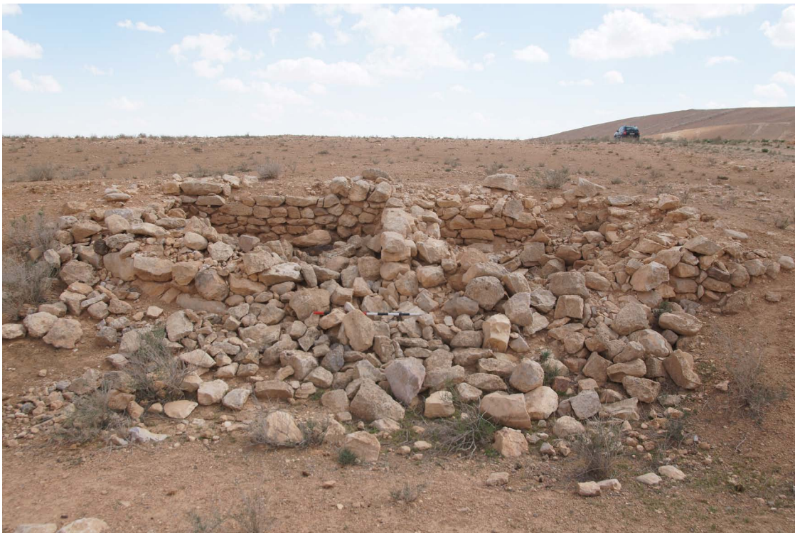
Building 209 seen from the N.
