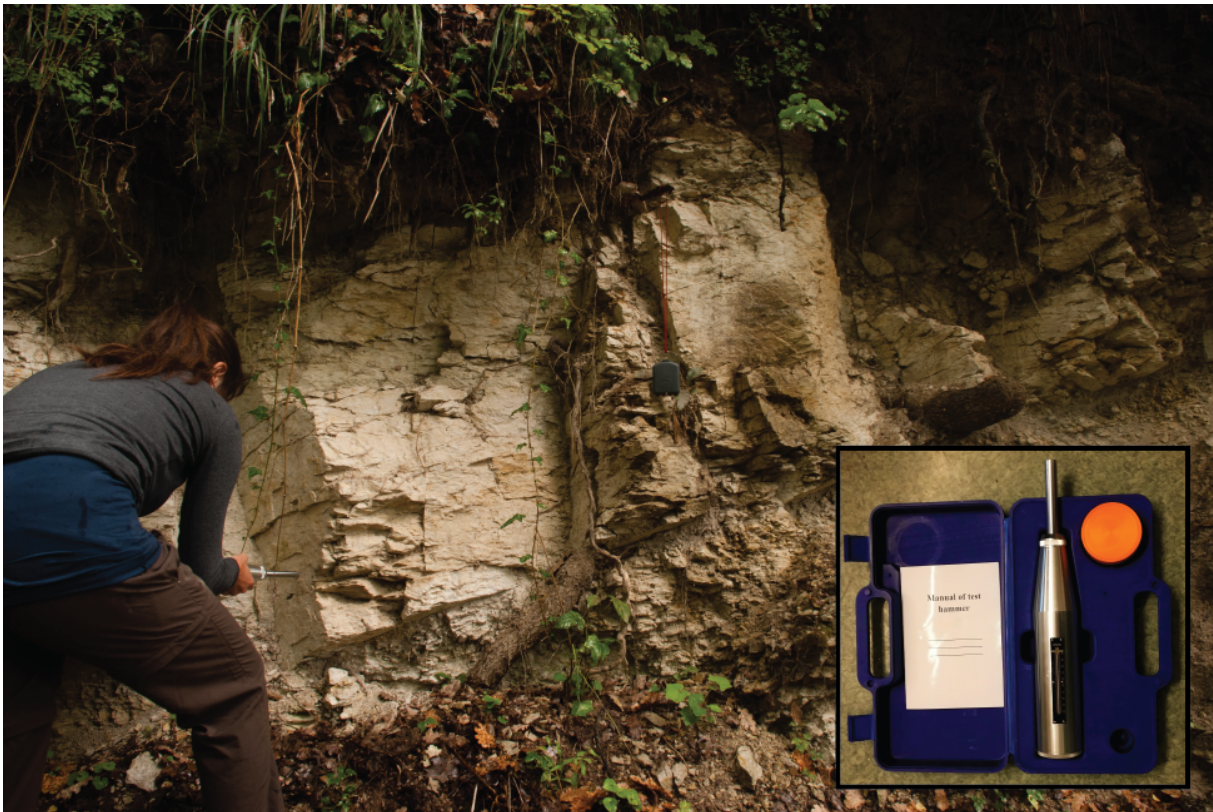
Fig. 11: Measuring rock mass strength by use of a Schmidt hammer can be useful to determine for example rock type and erosiveness. The instrument is shown in the lower right corner, and the procedure is illustrated on the main photo. By pressing the Schmidt hammer perpendicularly onto a surface, a pulse will emit into the rock, and the reflected signals are interpreted by the device to provide the rock strength value.
