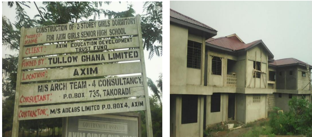
Plate 7: Axim Girls Senior High School dormitory under construction.
