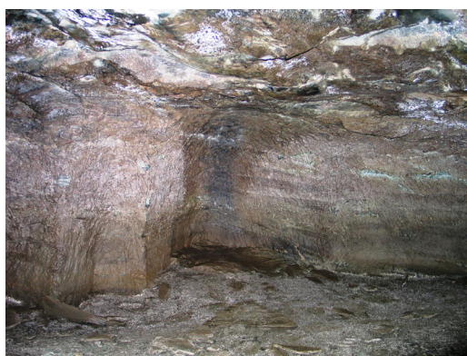
Figure 15. At Mannahidleren chlorite schist quarry, a large underground quarry, the walls display tool marks made by heavy iron picks, typical of exploitation of rectangular ashlars. (Photo: Ø. J. Jansen).
