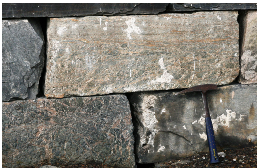
Figure 5. Onarheim church. Two soapstone ashlars (s) with a bluish tint displaying a brecciated structure, with veins of talc and carbonate. The upper half of the stone above the hammer demonstrates how the massive, lower part has been transformed to rock with well-developed foliation. (Photo: Ø. J. Jansen).
