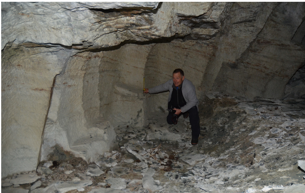
Figure 5. Carving traces in the underground quarry at Bakkhidlaren indicating extraction of tiles and slabs, possibly for building stones. (Photo: A. O. Martinussen).
