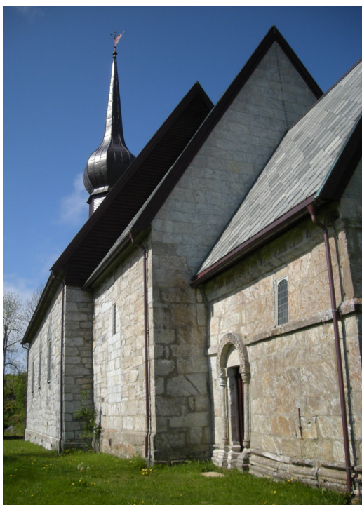
Figure 4. The medieval church at Alstahaug as it appears today after the rebuilding in the 20th century. To the right are the south walls of the old chancel and nave, built of soapstone. (Photo: B. Berglund).
