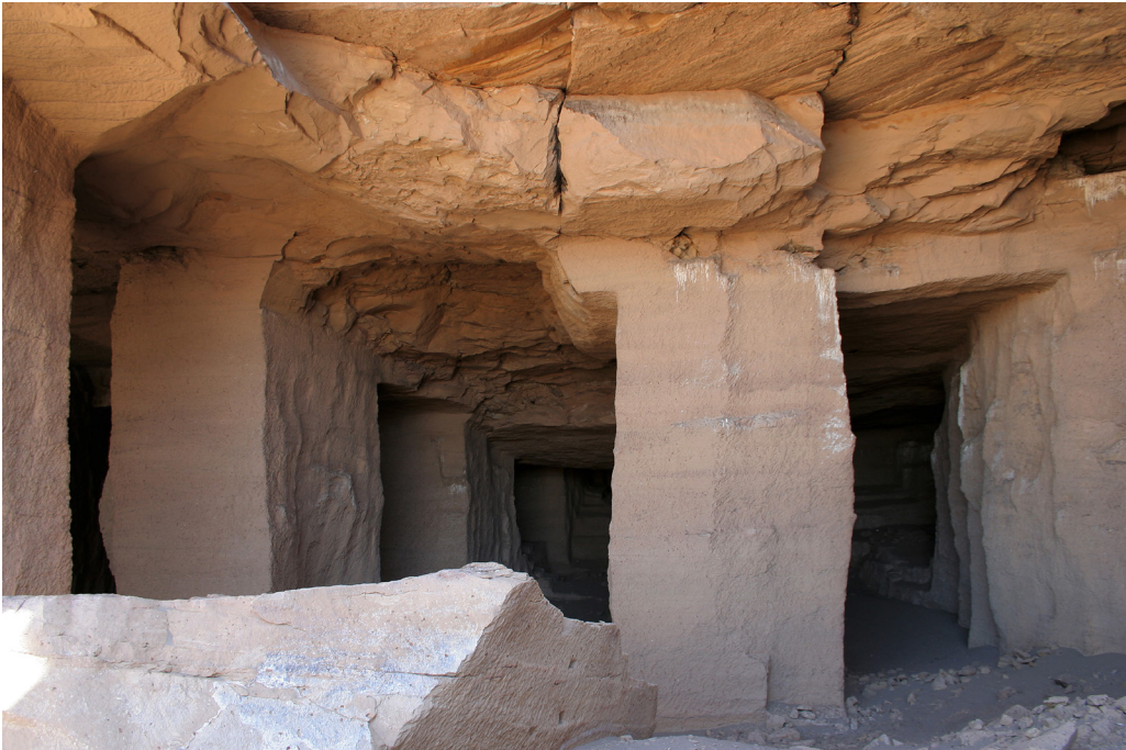
Figure 14. Typical ancient gallery quarry with pillars supporting the roof from caving in, here from New Kingdom Egypt (Gebel el-Silsila, Upper Egypt, c. 1500 BC). (Photo: T. Helda).
