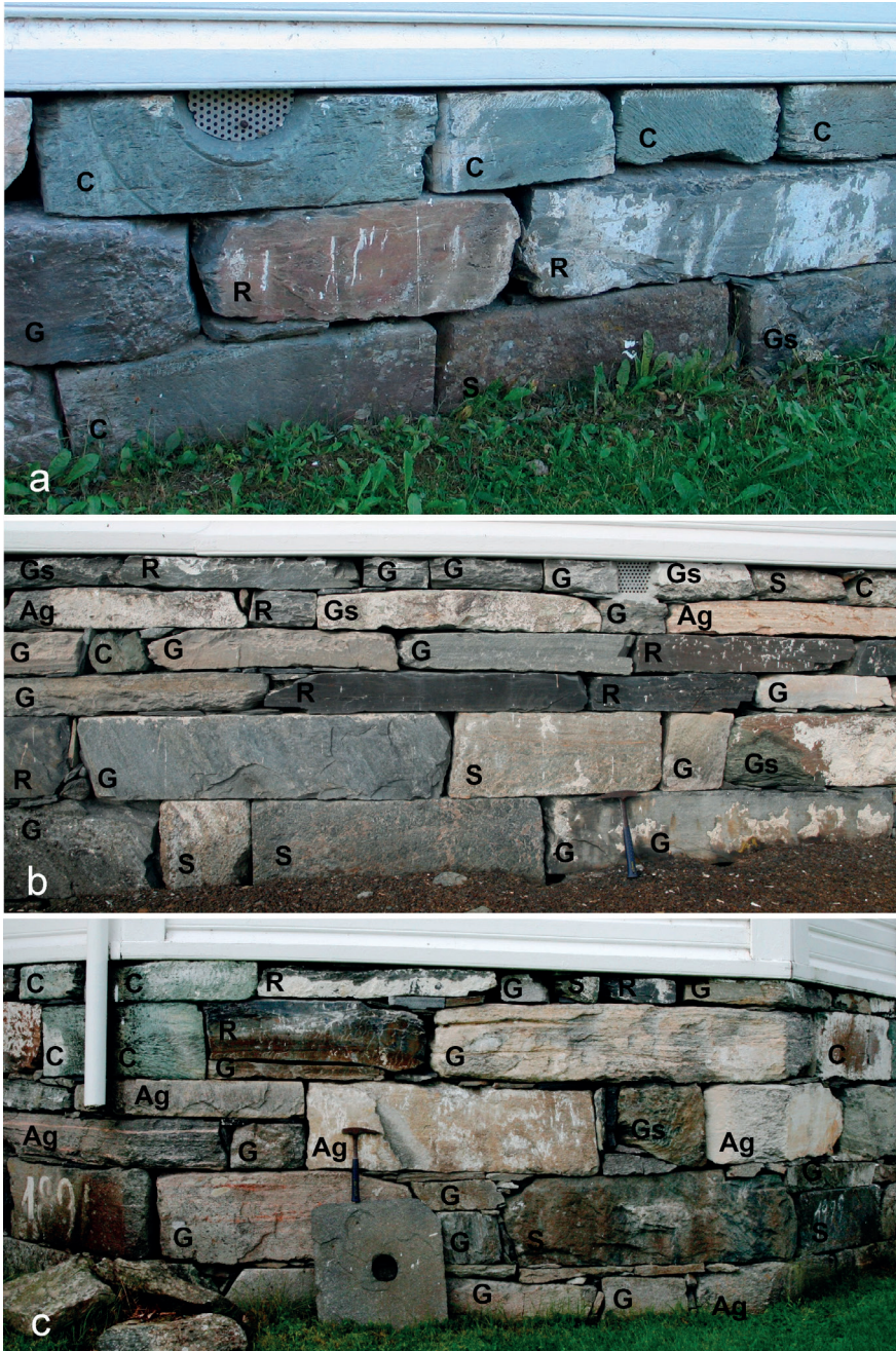
Figure 2. (a) Ashlars from chlorite schist in the upper course of the western foundation wall. Note the reused Romanesque window frame. (b) Ashlars of soapstone set in a coursed dry stone wall of undressed slabs and rubble. (c) Coursed dry stone walling in the north eastern part of the foundations displaying large blocks of mainly gneiss, however in the upper left corner are a few ashlars of chlorite schist. Legend: C = chlorite schist, S = soapstone, Ag = augengneiss, G = gneiss, Gs = greenschist, R = rhyolite. (Photo: Ø. J. Jansen).
