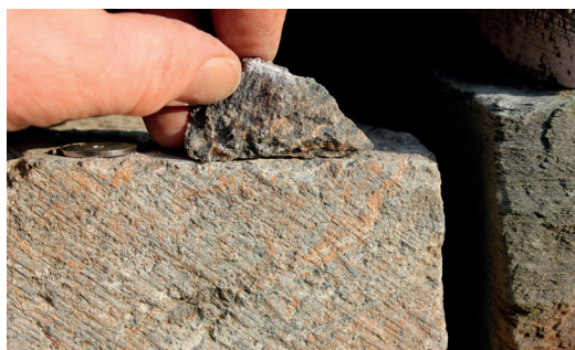
Figure 7. Small soapstone ashlar in the western foundation wall of the Onarheim church displaying a medium-grained mosaic of talc, carbonate and chlorite. The small piece above, sampled for analysis, shows the difference between weathered and un-weathered surfaces. (Photo: Ø. J. Jansen).
