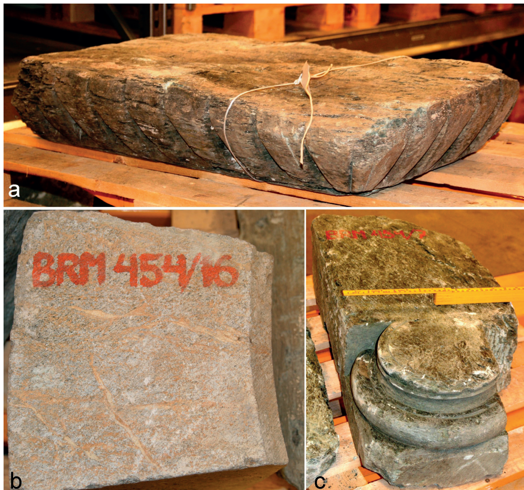
Figure 3. The University Museum of Bergen Collections: (a) Scalloped capital of chlorite schist; (b) Dressed block of soapstone; (c) Pillar base of chlorite schist. (Photo: Ø. J. Jansen).
