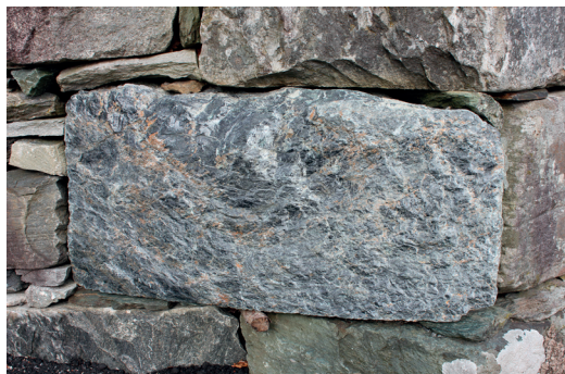
Figure 6. Soapstone ashlar with bluish tint in the dry walls surrounding the Onarheim churchyard. The ashlar was (re) worked parallel to the foliation, clearly displaying layers and lenses with chlorite, talc and carbonate. (Photo: Ø. J. Jansen).
