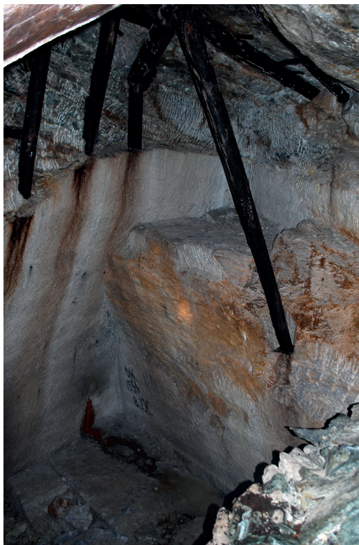
Figure 15. Early-modern underground soapstone quarry for production of soapstone ovens at Bagnes by Verbier in the Swiss Alps. One of the halls that can be accessed by a narrow adit, several tens of metres from the surface. (Photo: P. Storemyr).
