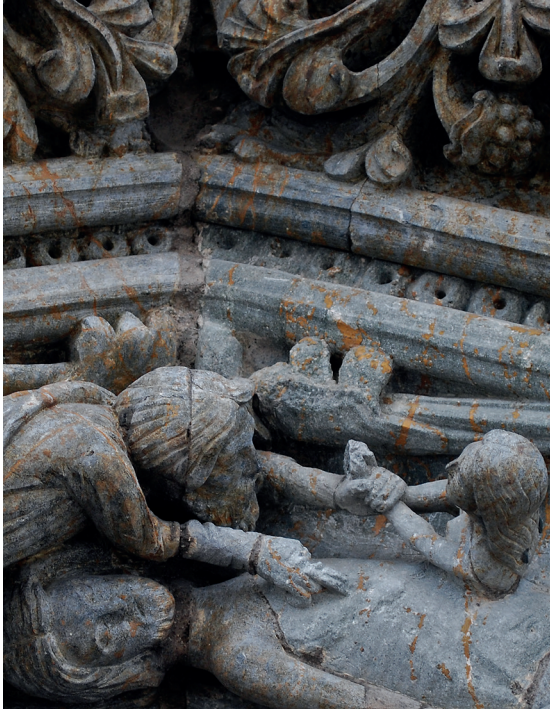
Figure 3. Trondheim soapstone used for intricate carving of a central Christian myth; the creation of Eva from Adam's ribs. To be seen at the so-called King's Porch at the south side of the choir, Nidaros Cathedral (first half of the 13th century). The scene was heavily restored in the late 19th century using Trondheim soapstone. (Photo: P. Storemyr).
