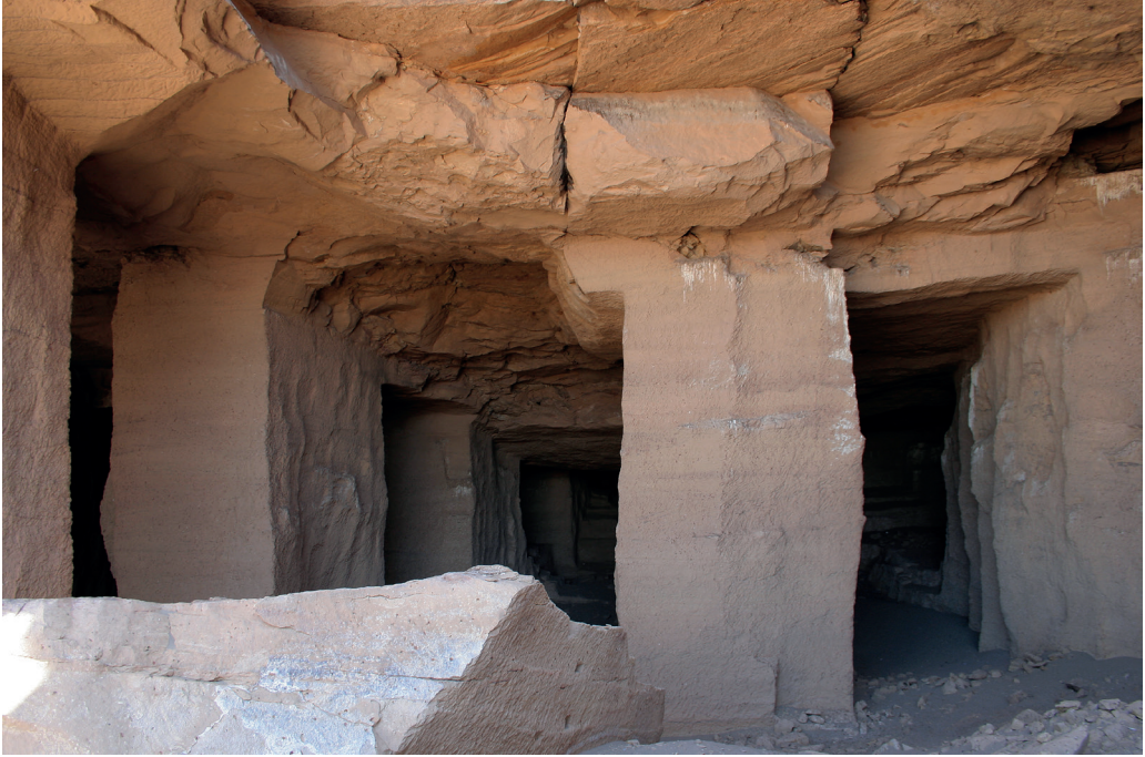
Figure 14. Typical ancient gallery quarry with pillars supporting the roof from caving in, here from New Kingdom Egypt (Gebel el-Silsila, Upper Egypt, c. 1500 BC). (Photo: T. Haldal).
