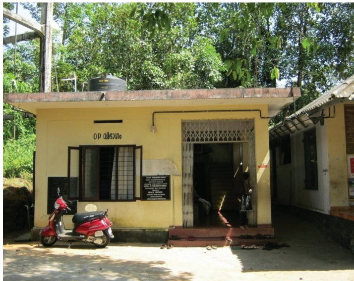
The newly constructed Out Patient wing at the Keranad Primary Health Center
