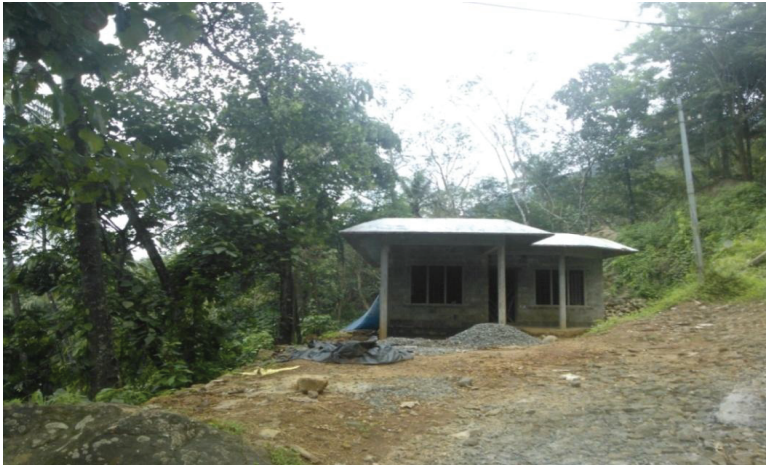
A concrete house under construction in Keranad during July 2013
