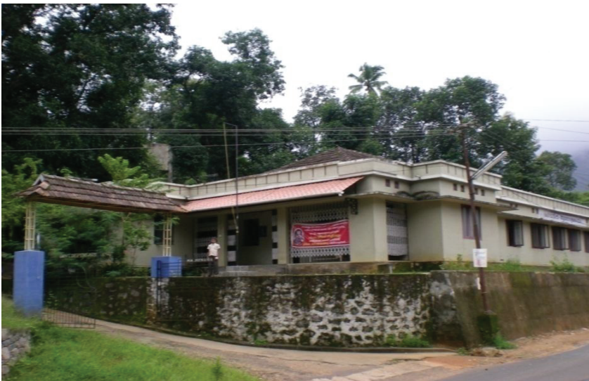
Keranad Primary Health Care center – a road side view
