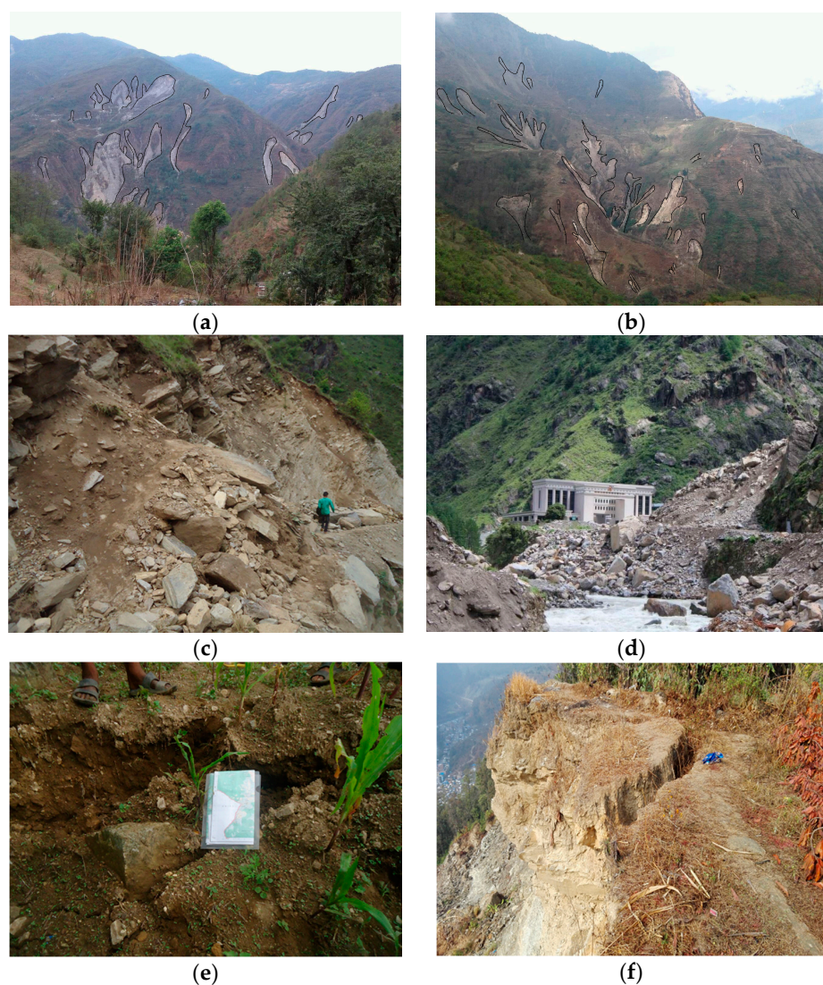
Figure 3. Co-seismic landslides observed during field survey: (a,b) landslides initiated on steep slopes; (c) rock topple; (d) rockslide partially damming the Bhothe Koshi at Rasuwagadhi; (e) observed cracking; (f) hanging block.
