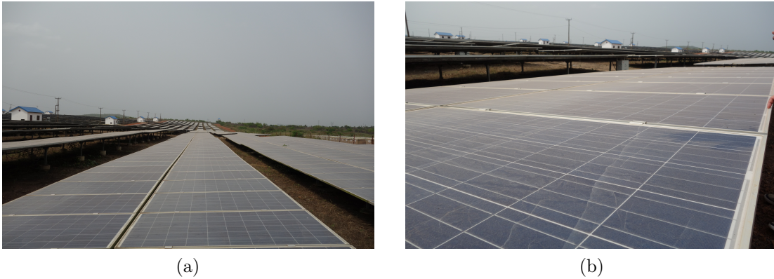
Figure F.3: Solar panels in the solar park in Onyandze covered with dust during Hamattan.
