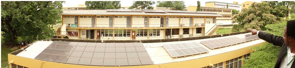
Figure F.2: The different solar installation at at the Department of Engineering at KNUST.
