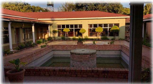
Interior courtyard of the ombudsman office building, as seen from the lobby.
