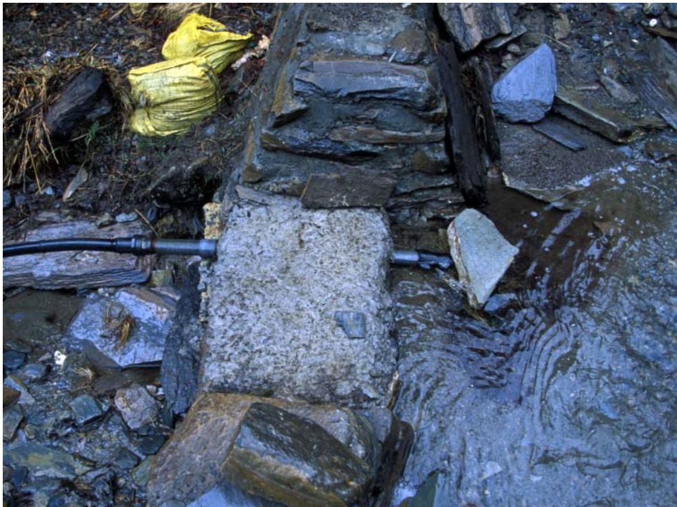
Pic 6.1: The drinking water intake in Ngawal. It is jammed by pine needles.
