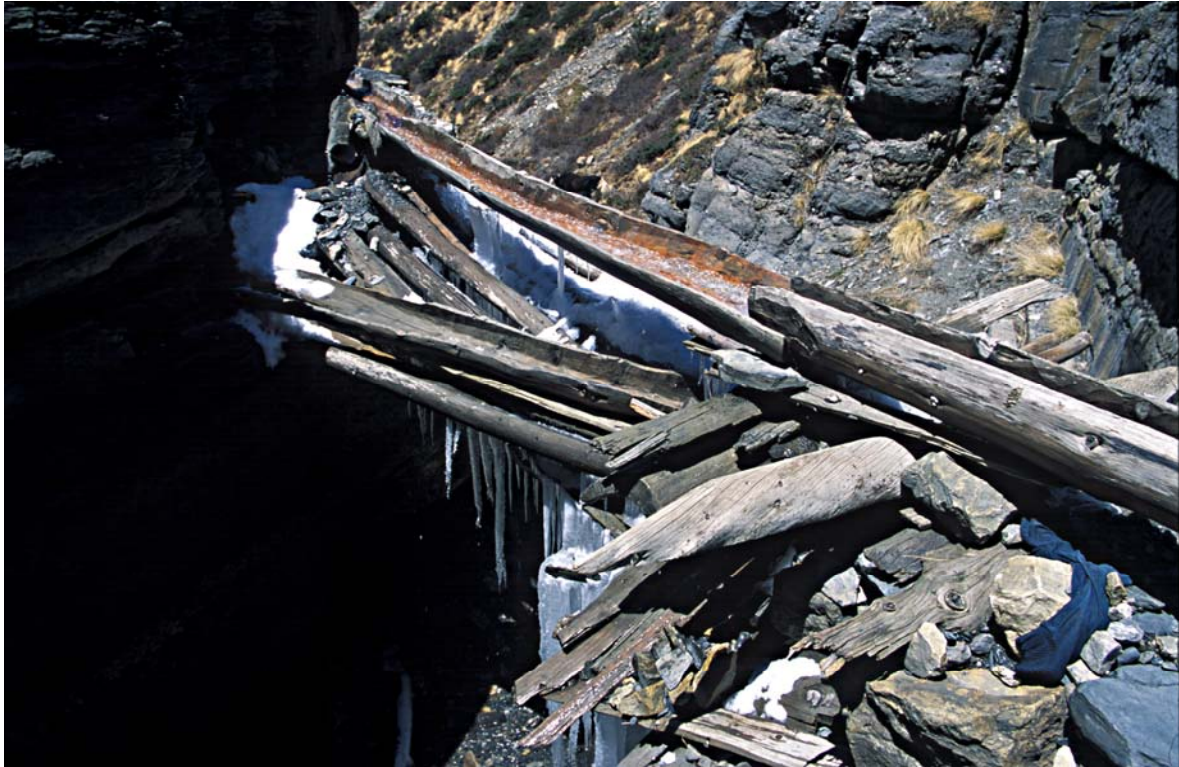
Pic. 4.1: Aqueduct made of wooden pipes at the start of the Teng Kyur pipe/canal. To maintain these kinds of structures is labour intensive, and requires well-functioning appropriation rules.
