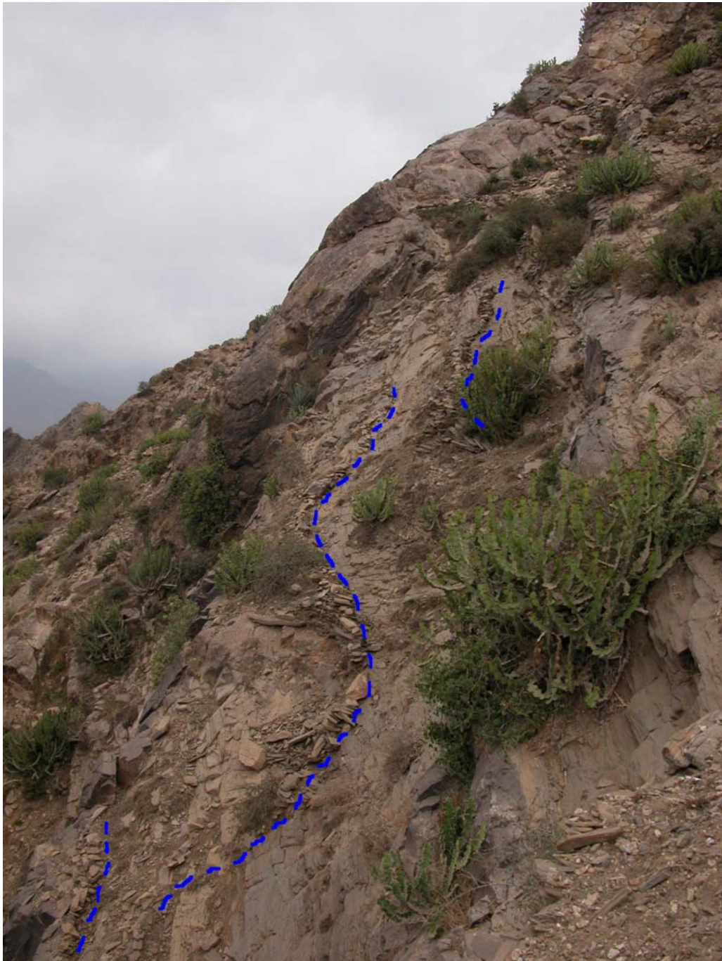
Fig. 14. The beginning of a minor collection canal. The potential water leading ability is indicated by the blue colour. The canal is very simply constructed by using rows and simple walls of stones as a guiding wall along the bare rock. When the water comes sand will partly fill the holes between the stones and make it more effective. This canal is very minor and is commonly used to guide runoff to agricultural terraces. This picture is taken in a low, eastern facing, dry area.
