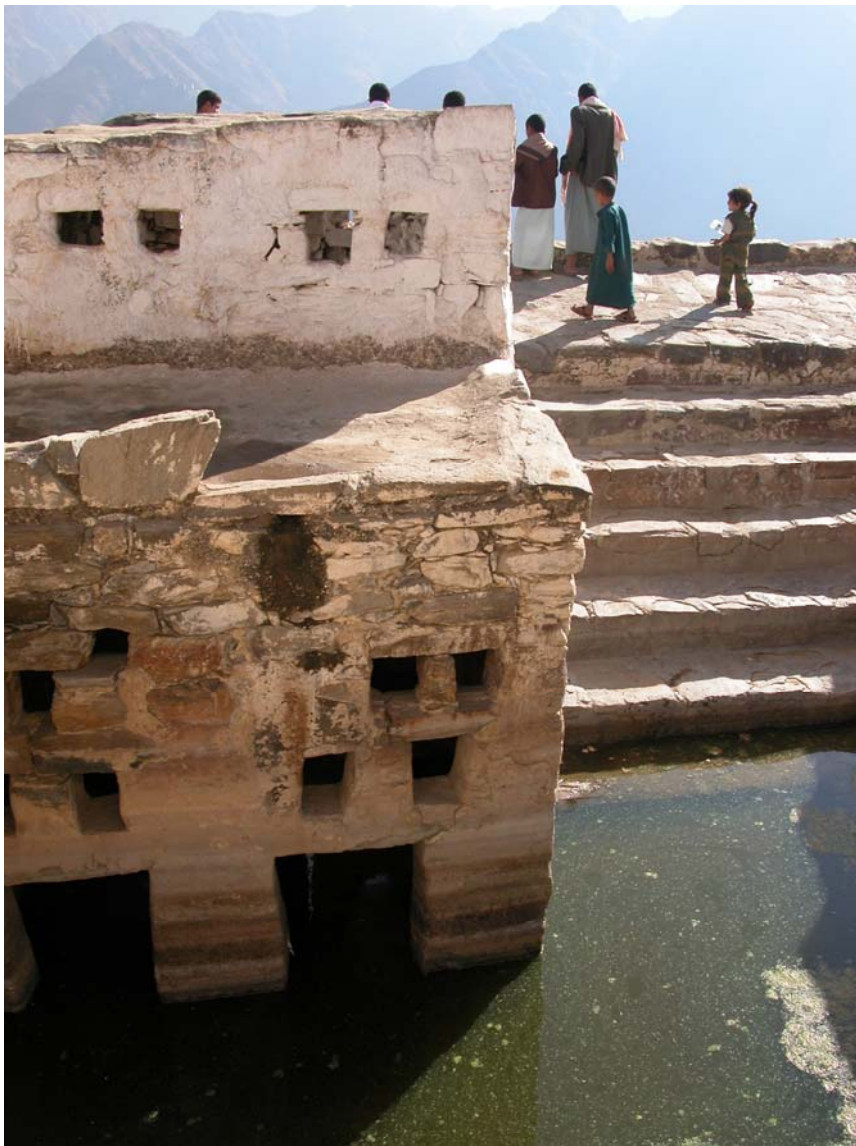
Fig. 22 Mosque cistern at Jabal Sidi. As there is no piped water here, the cistern is still used in a traditional way. The two “tunnels” leading down to the water surface are used when descending the stairs to perform the ablution in a private setting at varying water levels.
