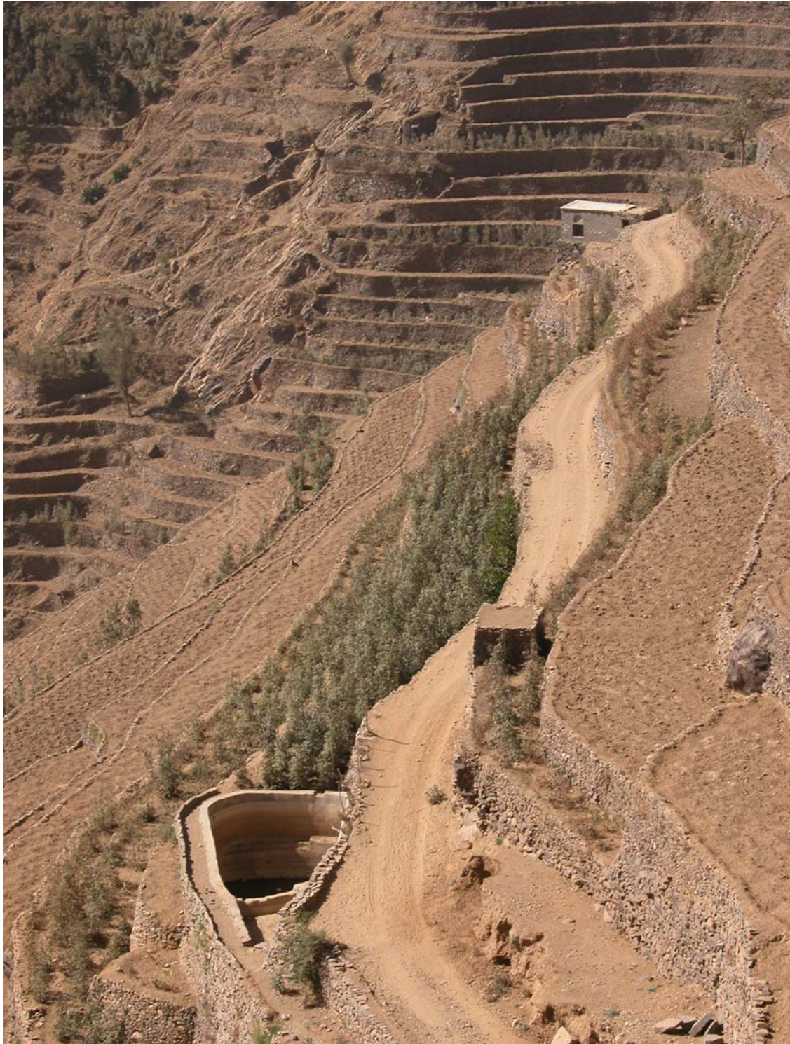
Fig. 23 Medium sized new private cisterns for qat irrigation. The cistern irrigates the qat that can be seen adjacent to it. The water is collected along the road toward the cistern and through the settlement basin in the end closest to the camera. The picture is taken during late spring before any heavy rain could fill it. The small houses are guard rooms as the crop is guarded from thieves during night, even close to villages. The water has to be pumped by a small portable petrol pump to irrigate all but the lowest terrace as the cistern is located at the same elevation as the terrace closest to the road. Such a cistern might cost 1.000.000 YR i.e. circa 5000 USD, but a price two to three times as much is also common. This picture shows a very well performed integration of a car road into the traditional landscape. Very often, walls are not resurrected and the masses that are left over from the construction, just pushed down the side. Restoration of terraces is usually only seen in conjunction with qat
