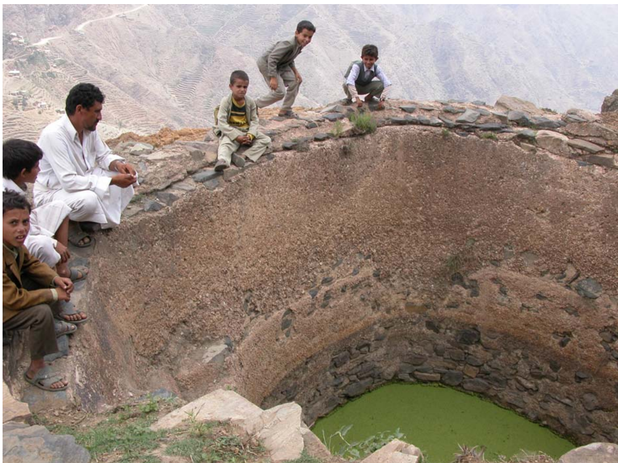
Fig. 30 Talking with a farmer on Jabal elbrith, Himla. Different layers of qadad can be seen as the water has throughout history etched the qadad away and new layers have been added. In the lowest part one can even see the masonry behind the qadad. According to the farmer, the cistern was in need of repair as it was leaking too much, especially when more than half full. Note the layer of floating plants, probably a type of duckweed.
