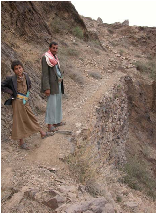
Fig. 15 Left: A major collection canal passing an aqueduct and can be seen extending upwards with a steady inclination. If collection canals are strongly built, it is common to use them as roads passing by otherwise steep sections. Here, it can easily be seen that it needs to be cleaned out and made deeper if it should convey more than a very small flow. The outer edge gets worn by people and animals.
