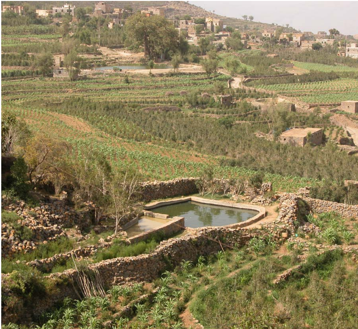
Fig. 25 Below: Private cistern in Mabyan. The runoff is from a public road, one can see that the water in the settlement basin is yellow of colour and quite clear in the main tank.
