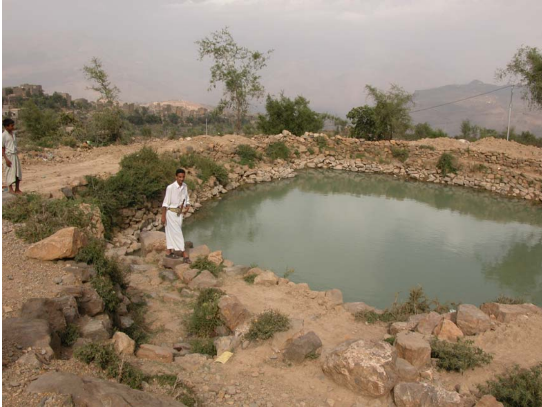
Fig. 19 A mansuriyya type cistern between ʿAjrama and Bayt Shamah in Mabyan. It was said to be 7-8 m deep and it is somewhat wider than that across. Note the complete absence of plastering. The inlet canal is from the middle of the bottom line of the picture leading to just to the left of the man in white. The canal has a “step” down, close to the lower edge of the photo. This detail is called ʿatgala and is described in part 3.3.
