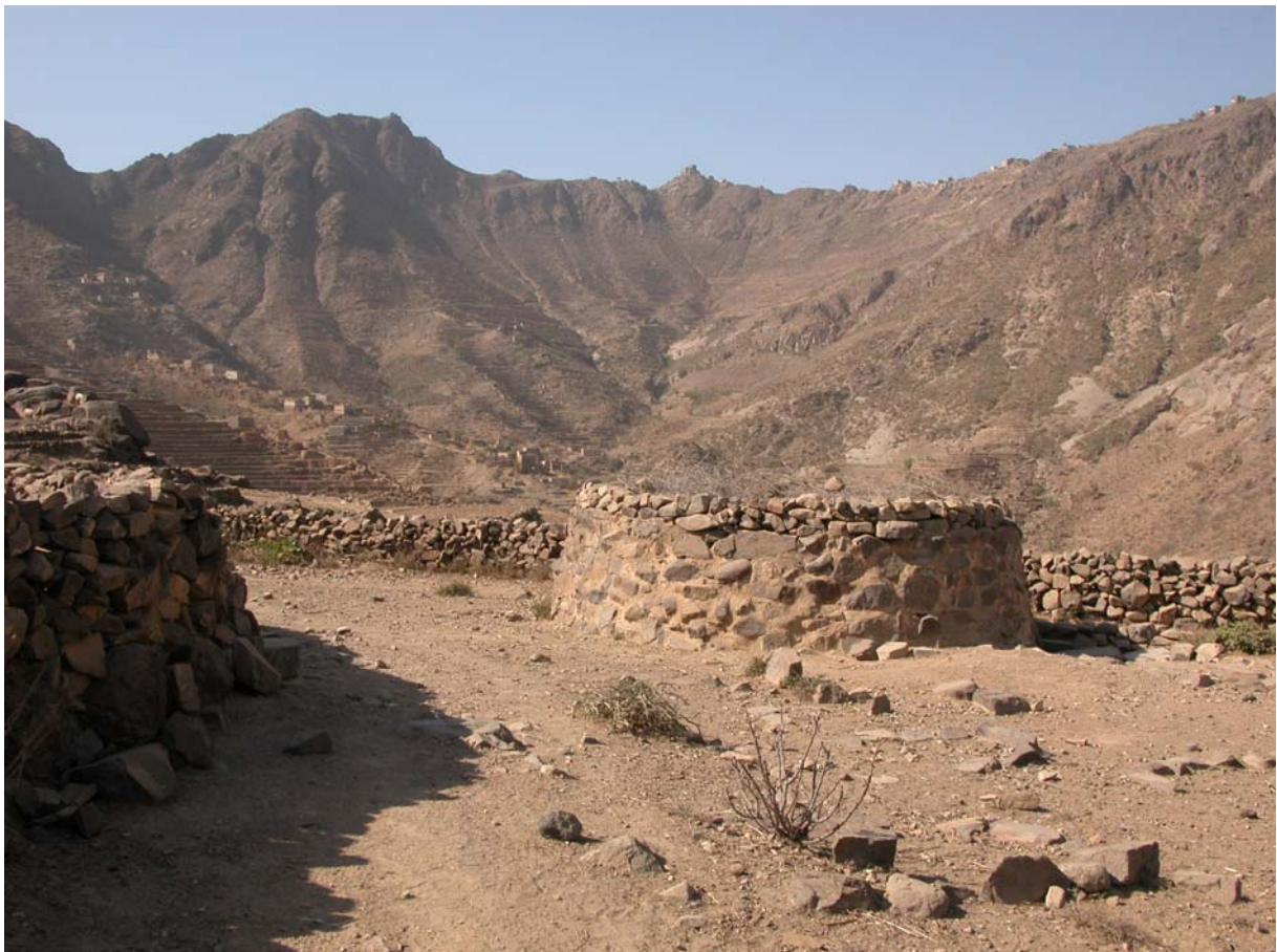
Fig. 38 The village of Dabbān in northern Bantalemsōit toward the south with an old qadad treated cover-structure over a cistern. Entering through a small door that can be locked, the cisterns look the same here as in Hajja. The covering structure is made with cantilevering masonry with qadad between the stones. The internal
