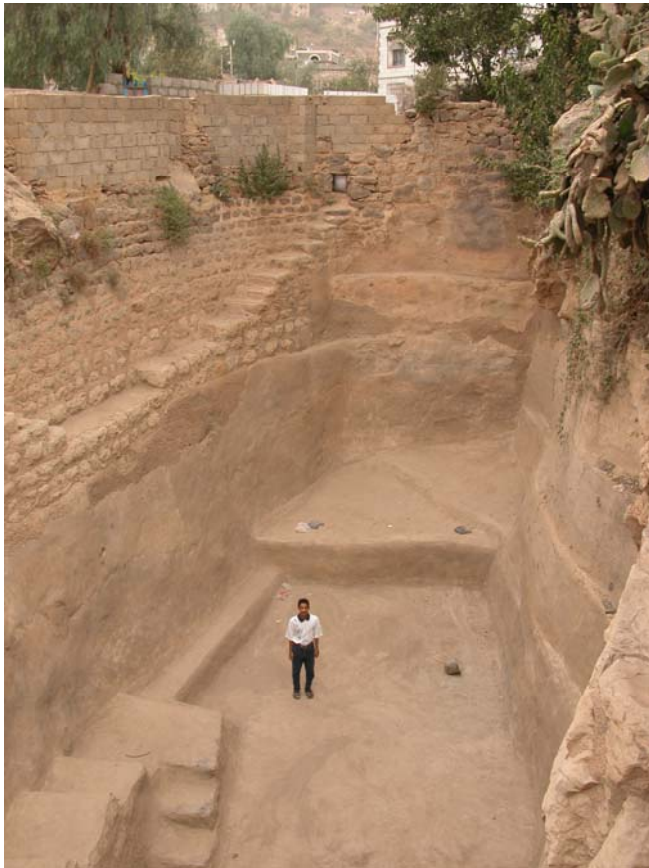
Fig. 20 Left: The cistern at the quarter of Hajja city called al-Qala'ā. The cistern is empty and has just been cleaned out. The water enters through the presently closed hole at the top of the stairs.
