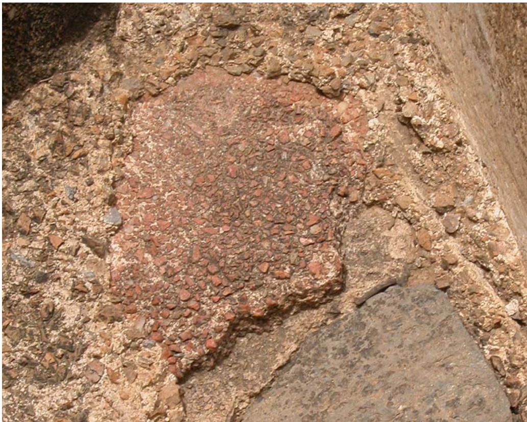
Fig. 29 The up-facing part of the rim of a cistern. Several thin layers can be seen, also with slightly different colours of the aggregate stones. The red part in the middle has probably been polished as one can see that all the aggregate stones are level and smooth. The aggregate stones are rarely larger than 1 cm.
