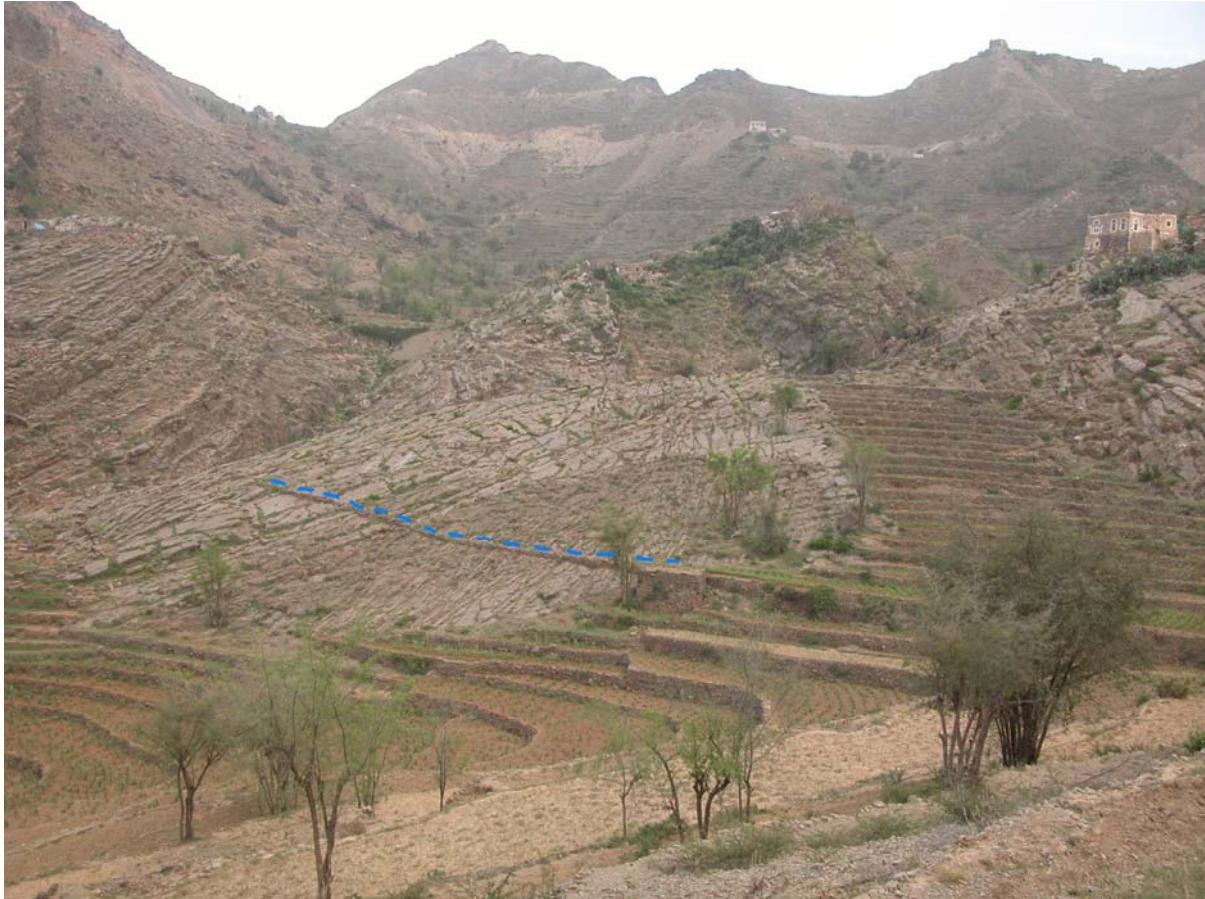
Fig. 8 A very clear stone made collection canal for supplementary rainwater harvesting. The fields in the picture rely on direct rainfall, but the collection canal increases the water supply. The first terrace receiving the extra runoff is clearly greener than the others.
