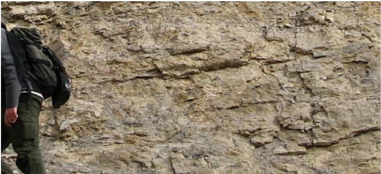
Figure 2.9 East-looking photograph beneath “17” in Figure 2.10. View of the Master Fault surface. The striated surface is exposed in a patch of 10 by 10 meters approximately. Weathering masked the original pattern over much of the exposure. Scale: photograph is about 1,5 meters in height. The strike and dip of the fault is 310/43 SW. The rock surface is broken and in places brecciated, attributed to fault slip. The fault slip may create the observed brecciation. Stereographic projection in Figure 2.13 (a-d).
