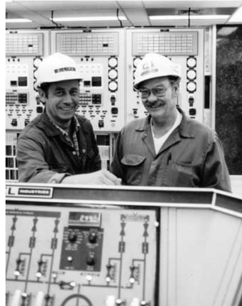
Figure 11. Process technicians in the control room in the 1970s. Photo: Norwegian Petroleum Museum.
