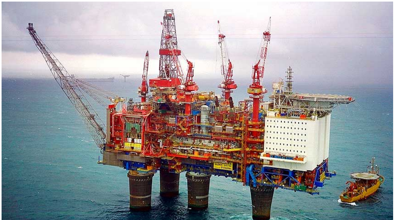
Figure 1. The oil platform Gullfaks A with its three main sections: the drilling area to the left with the characteristic derrick tower, in the middle; the process area; and, to the right, the white-coloured living accommodations with the helicopter deck on top. To the right a supply ship, and in the background a tanker is tanking oil. Photo: Statoil.
