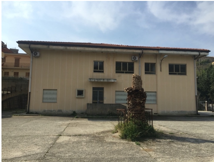
Photo 13: The office of CIR seen from the parking lot. By author.
