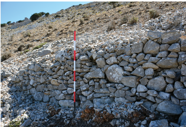
Figure 5. Photo showing an intact terrace wall acting as a barrier to erosion material from a collapsed terrace above. Note the large amounts of quarrying waste flowing over the terrace.
