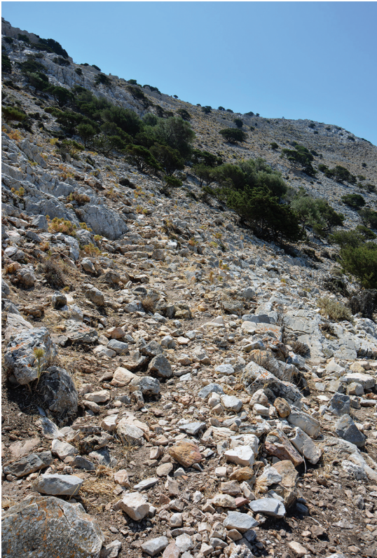
Figure 3. Photo showing a section of the terraced path (foreground) and a section of rock-cut steps (background).
