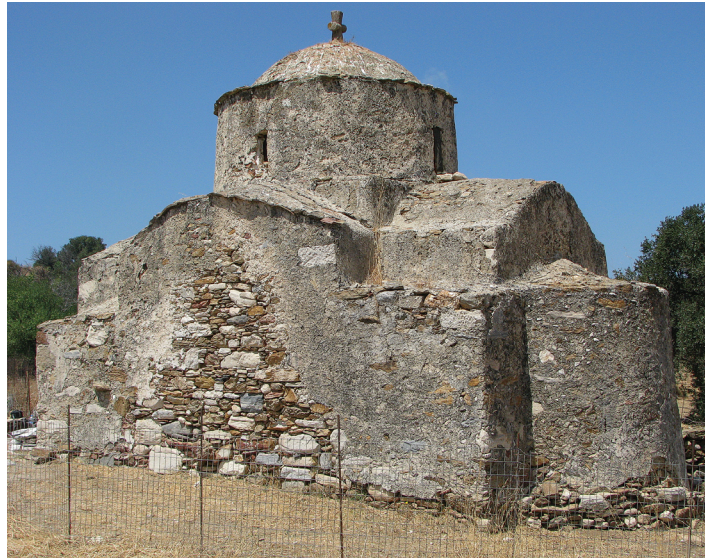
Figure 38. Christos at Kathanychta. Southeast view.
