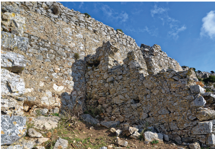
Figure 12. Cistern to the north of the stepped entrance with supporting buttresses added later when the structure was converted to hold a cistern (marked as B on fig. 4).
