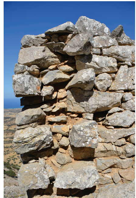
Figure 3. Photo showing clay/earth bonding within a wall and the light use of mortar on its external face.
