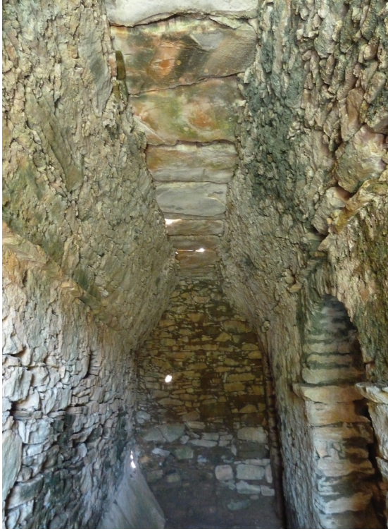
Figure 4. Naxos. Agios Isidoros Tragaias. The pseudo-vault of the narthex built in the corbelling technique.
