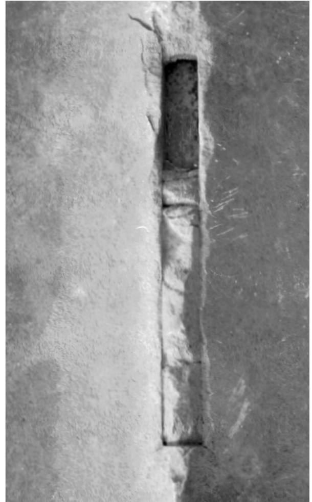
Figure 15. Arriis repair on the column drum 809. (Photo: Pakkanen 1995)
