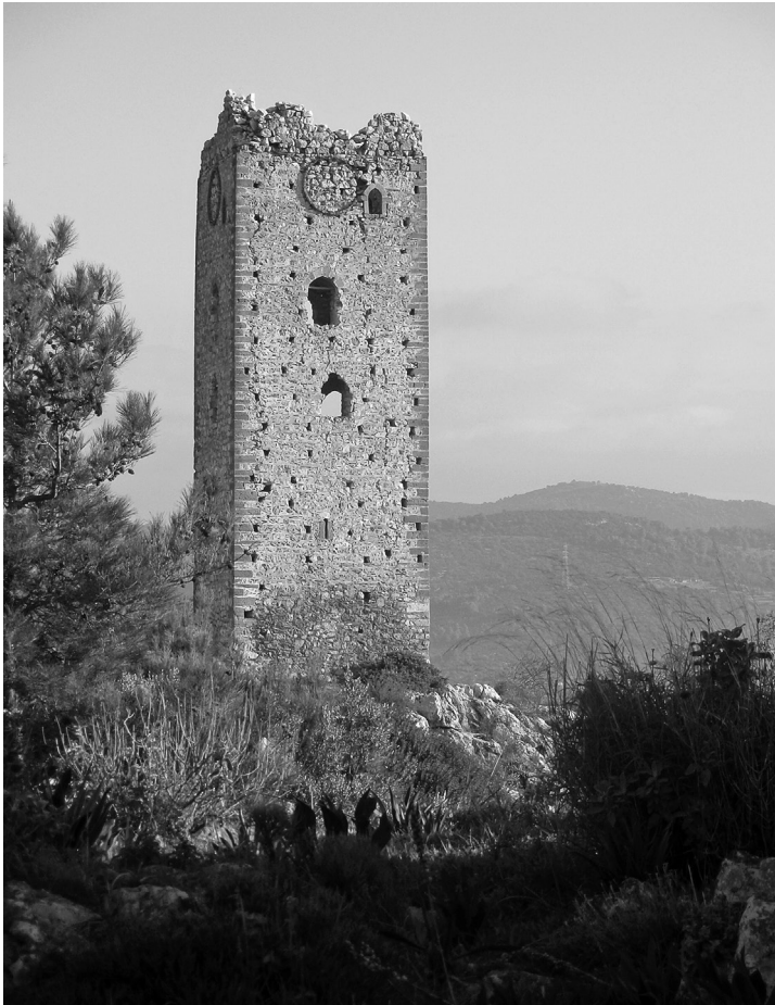
Figure 4: View of the south tower at Phylla, Euboea. South face (by the author).
