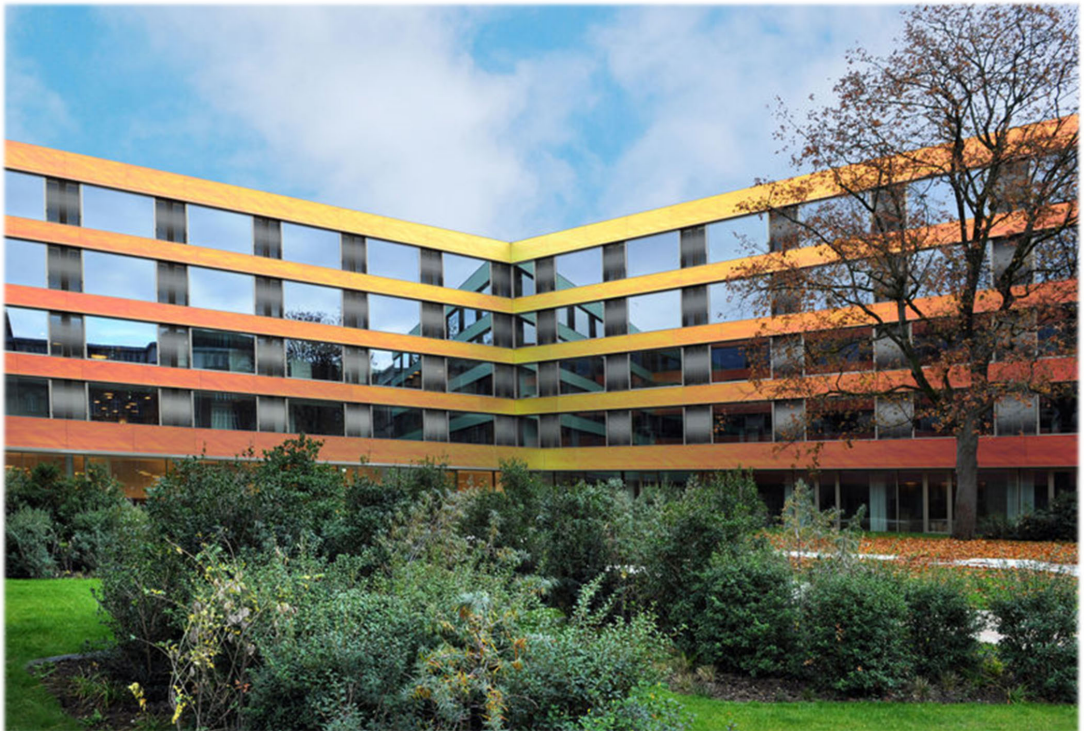
Figure 4: University Childrens Hospital Basel, Switzerland.
