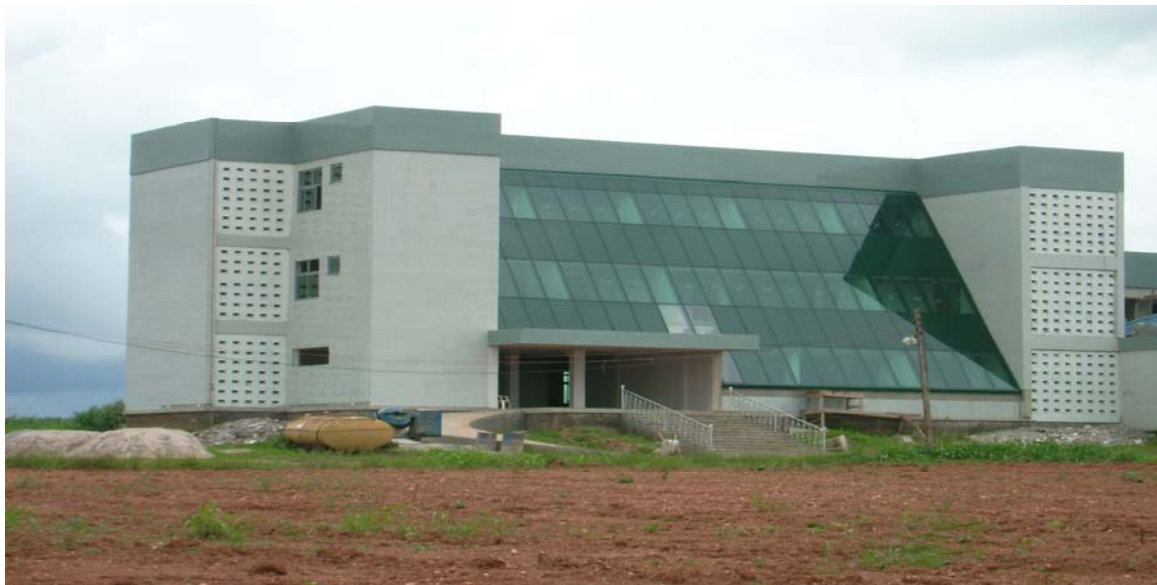
Picture 4: The uncompleted Administration Block of the Inland Port Project
